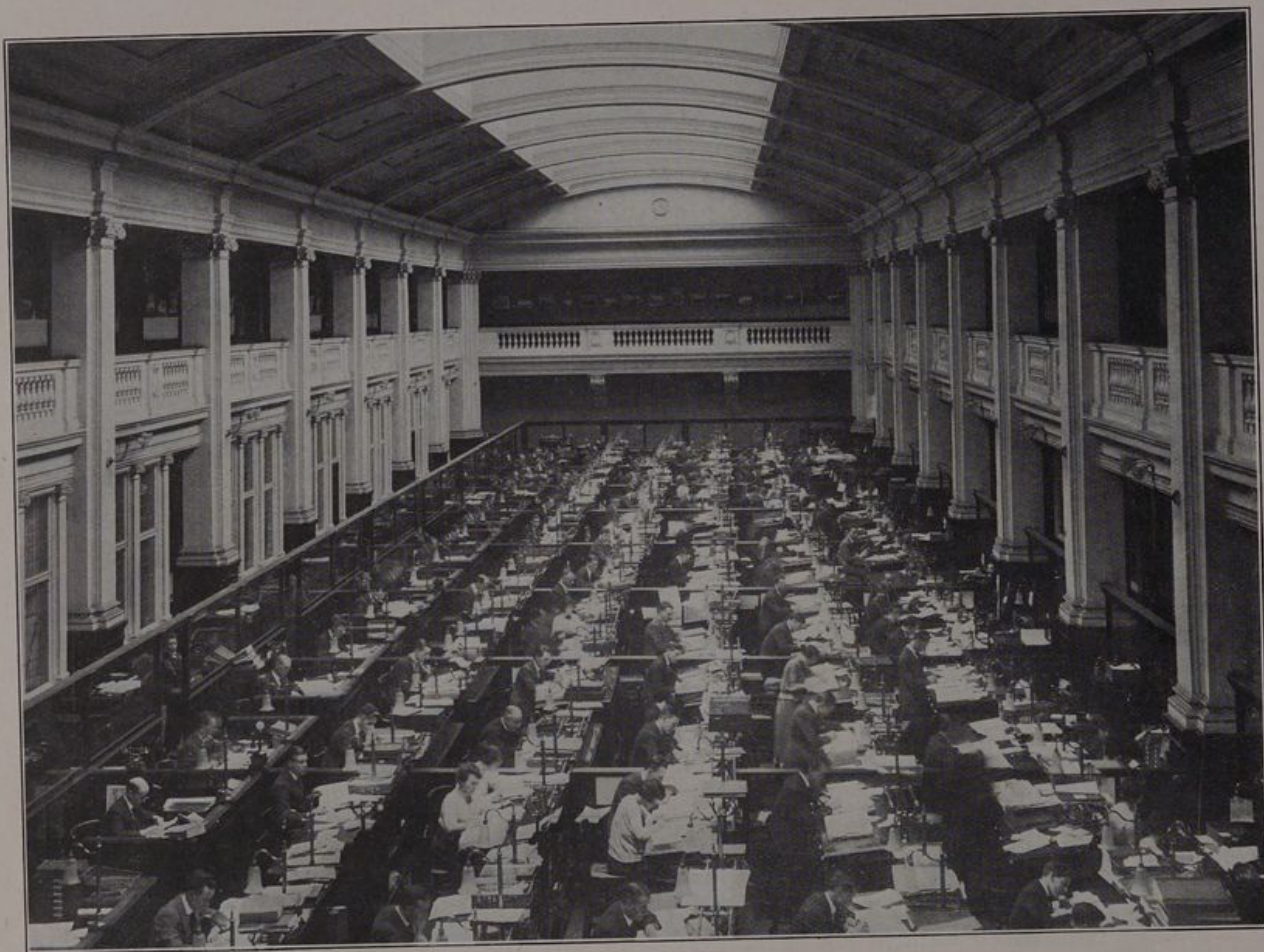
SOUTH WING OF THE GENERAL OFFICES
