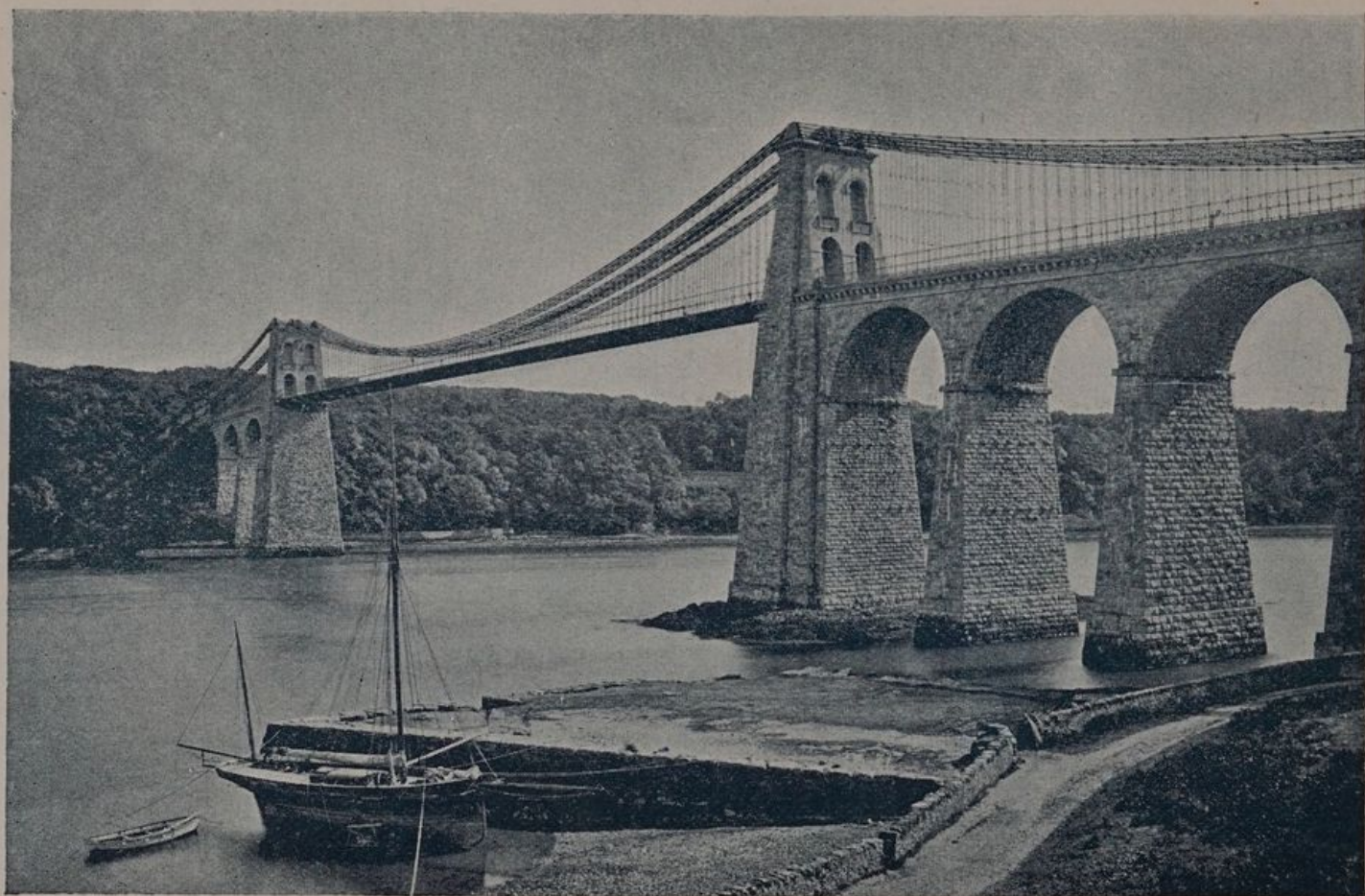
MENAI SUSPENSION BRIDGE.
