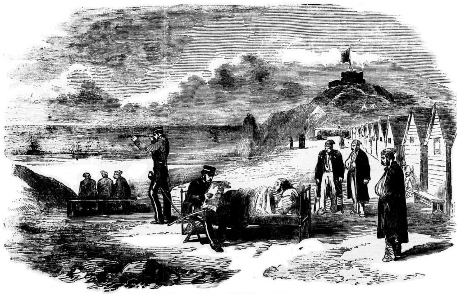
THE NEW CASTLE HOSPITAL, AT BALACLAVA.
