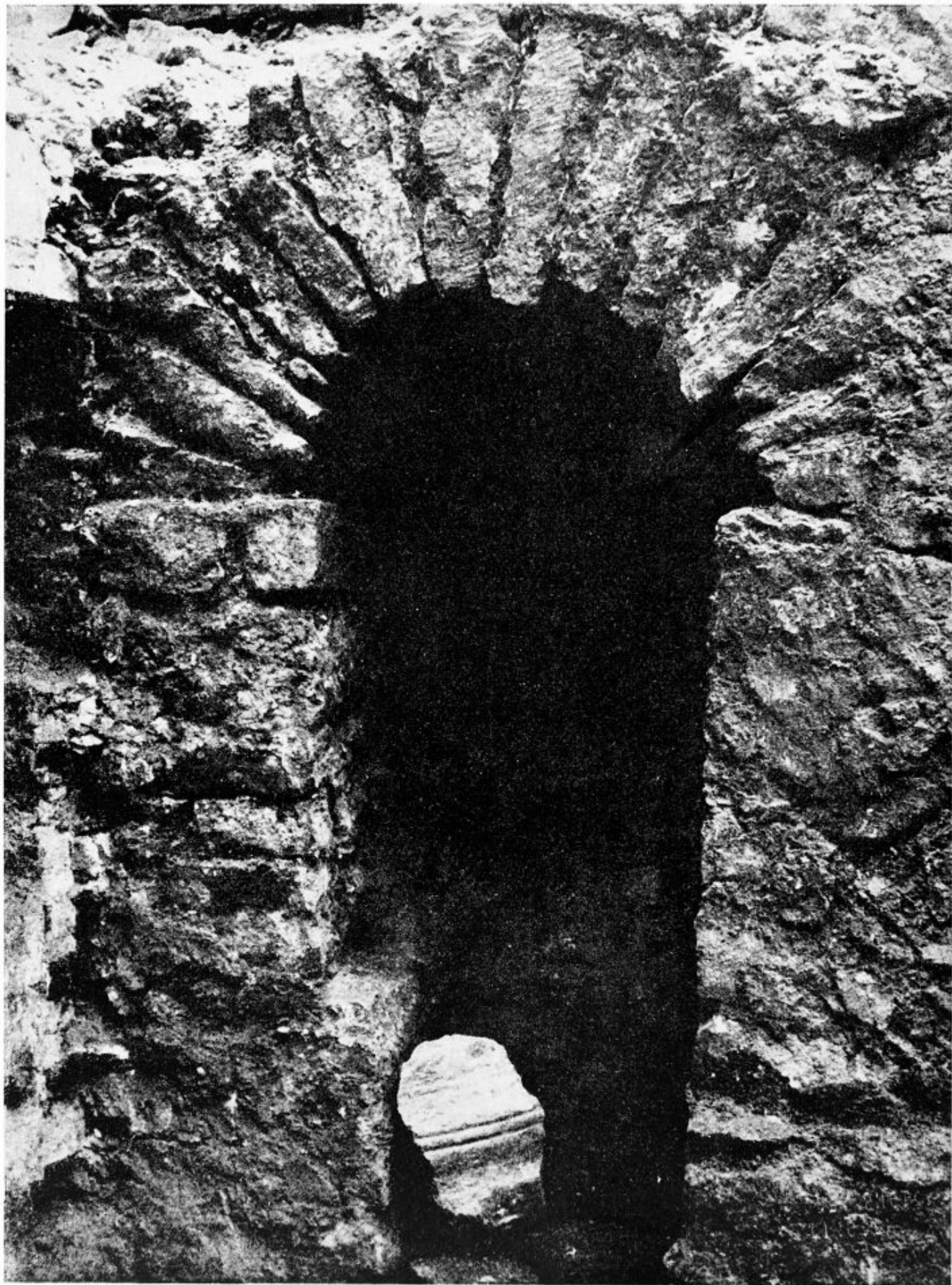
FIG. 28. LINCOLN. SEWER UNDER BAILGATE.
