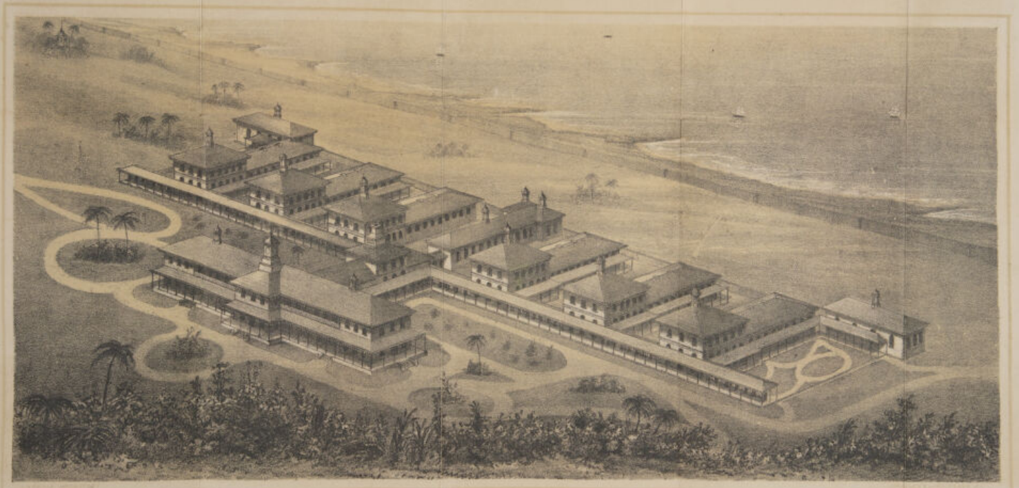
GENERAL VIEW OF CANALON REYSER
