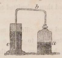
take one part of sulphuret of antimony of commerce, break it into pieces of half the size of split pease, put it into the flask, and pour upon it four parts of common concentrated muriatic acid (spirit of salt of commerce). Sulphuretted hydrogen gas will become disengaged from the materials in abundance, and pass through the water in the vial (c). Let the extrication of the gas be continued for about five minutes; and if the minutest quantity of lead be present, the
