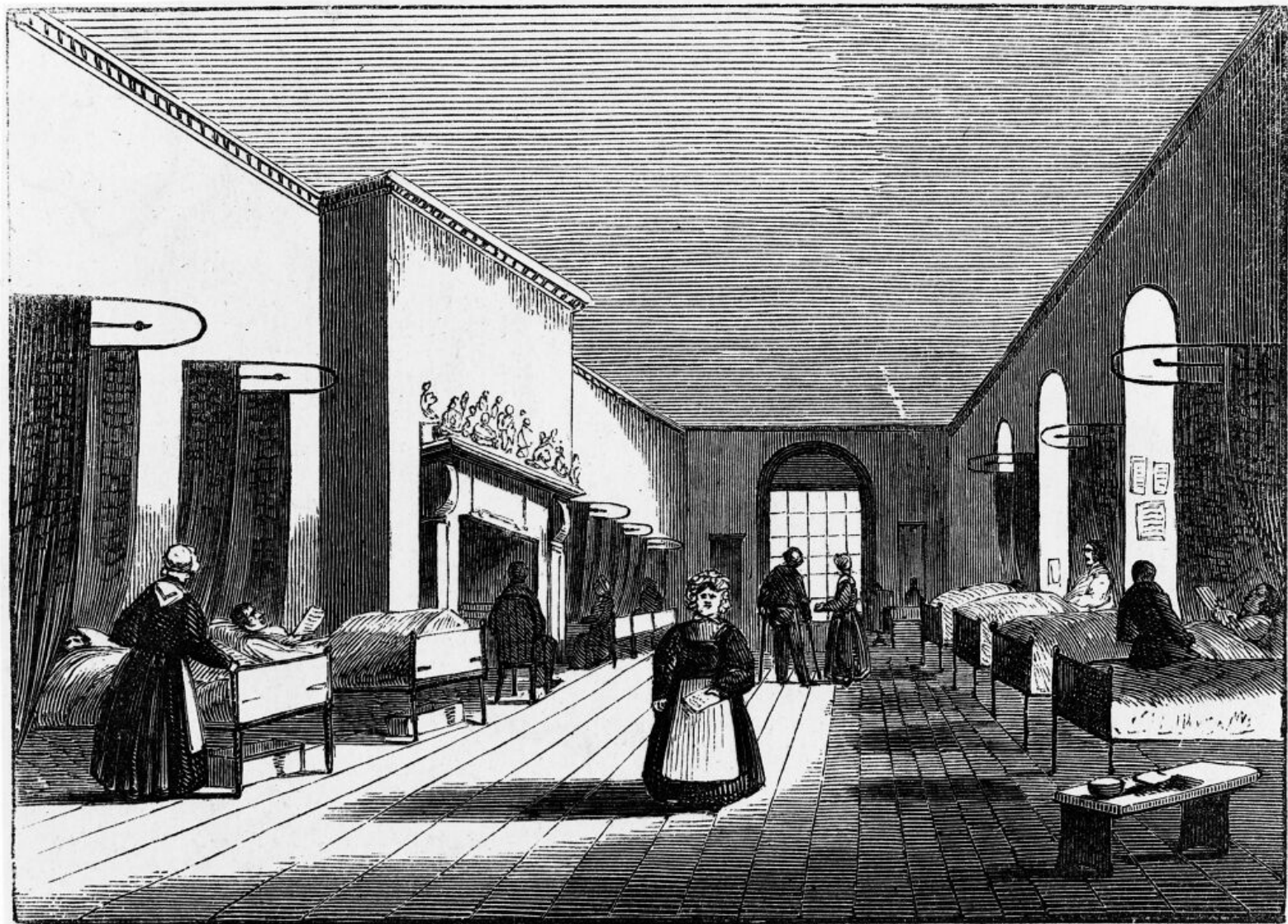
Interior of Rahere's Ward, St. Bartholomew's.
