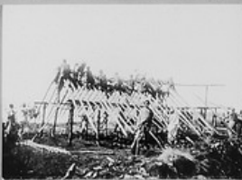
Erecting Hospital (barrack system)
