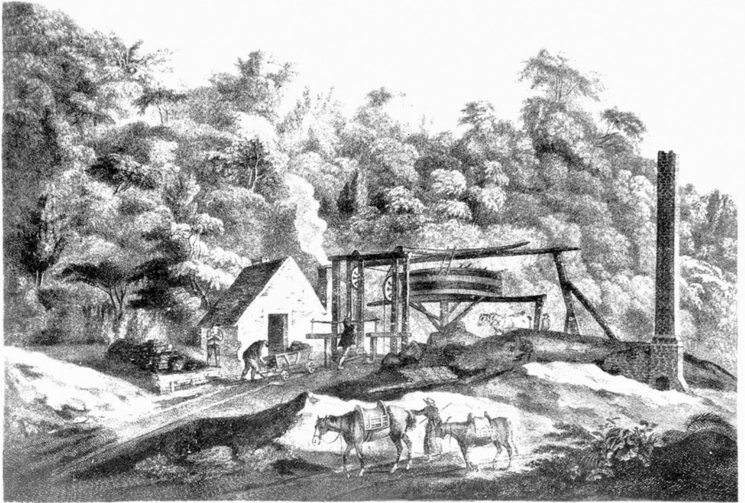
A Pit-head at Broseley in Shropshire. From: The King's Topography , British Museum.
