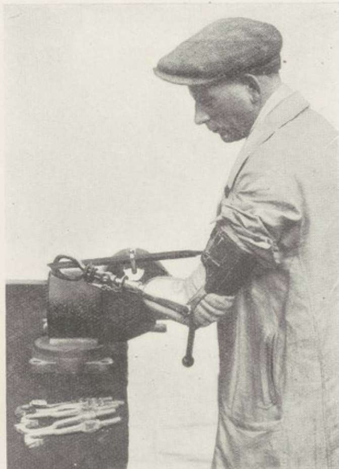
FIG. 158.—BLATCHFORD WORKER'S BELOW ELBOW ARM IN USE WITH BOND'S HOOK.
