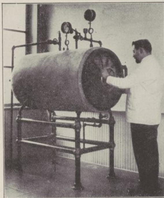
This sterilizer, in Research Laboratory, Johnson & Johnson, is piped exactly as shown in Fig. D.
