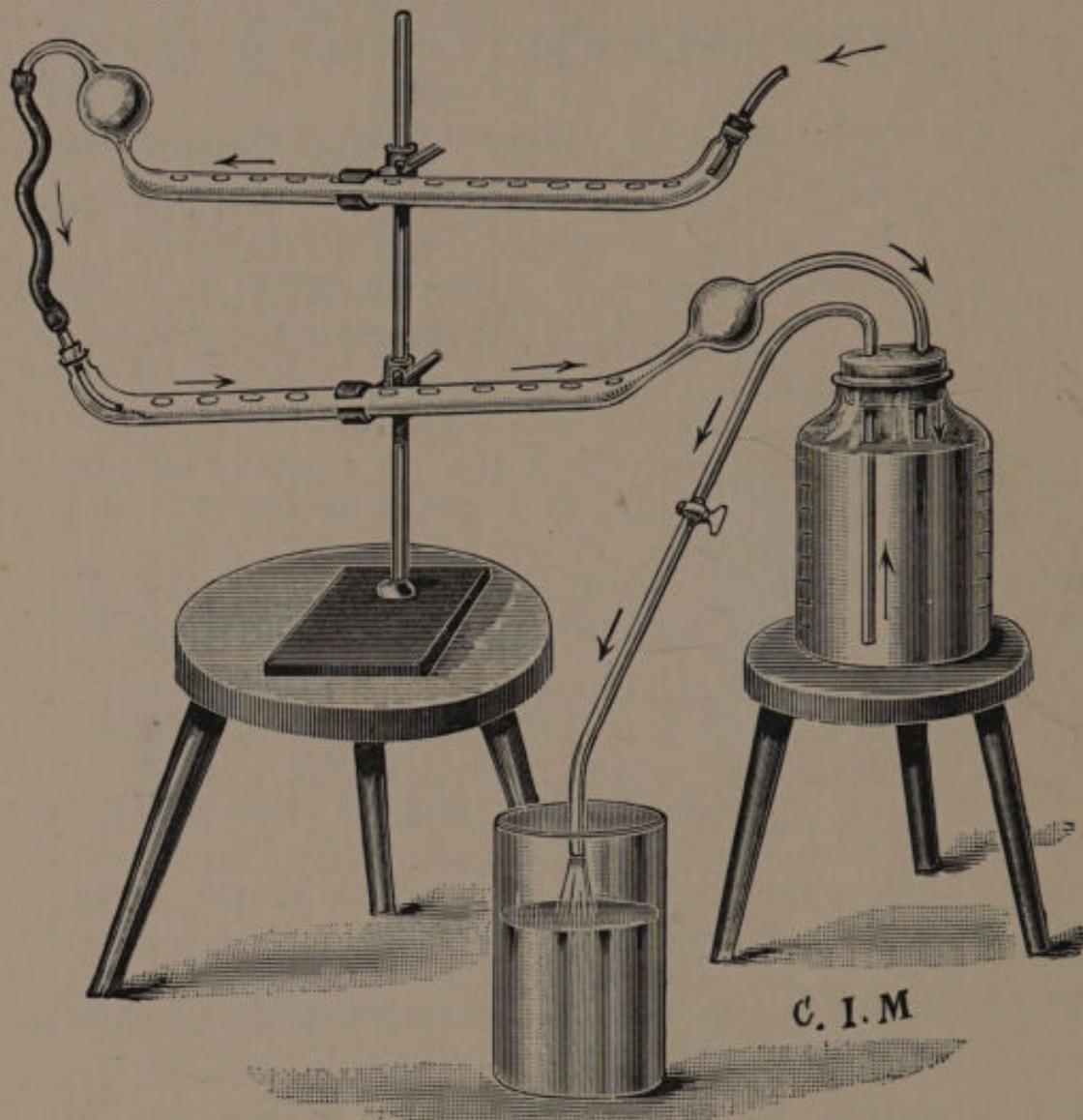
FIG. 19.—Estimation of  $\text{CO}_2$  by Pettenkofer's Tubes.
