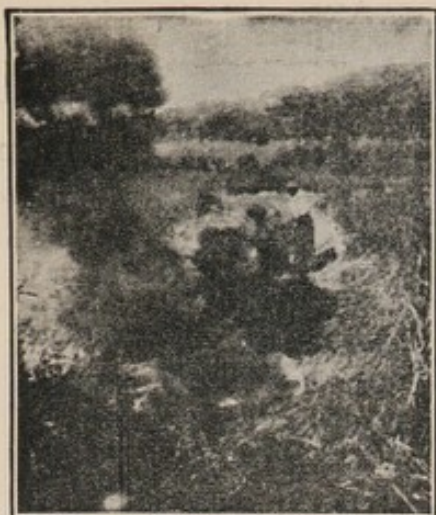
FIG. 60.—Vegetation along the side of drainage ditches may be easily burned if saturated with crude oil.
