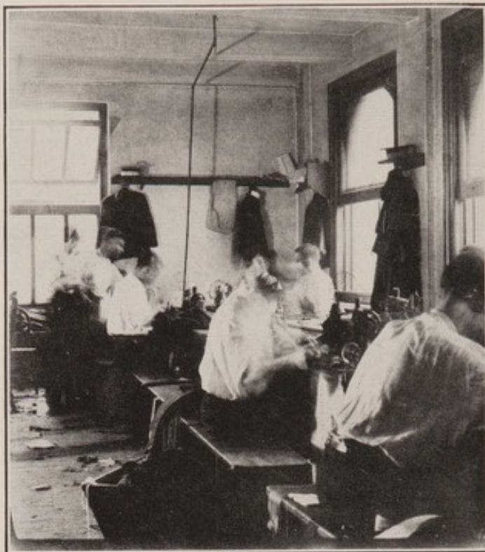
Fig. 3.—Fish-tail burners used in the illumination of machines. The flickering of the flame and the glare from its proximity to the eye make this form of artificial illumination very undesirable.
