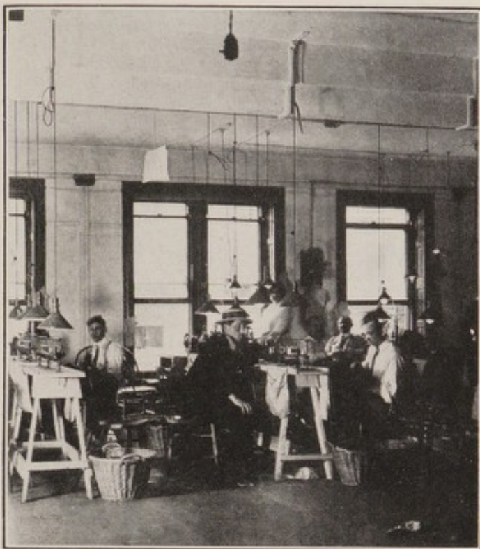
Fig. 5.—Finishing tables. Lamps project below reflectors. The daylight illumination was good.
