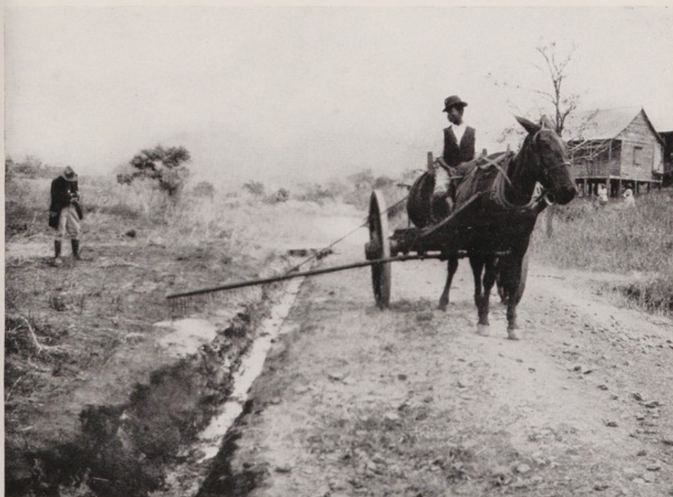
Oil cart for applying oil to roadside ditches
