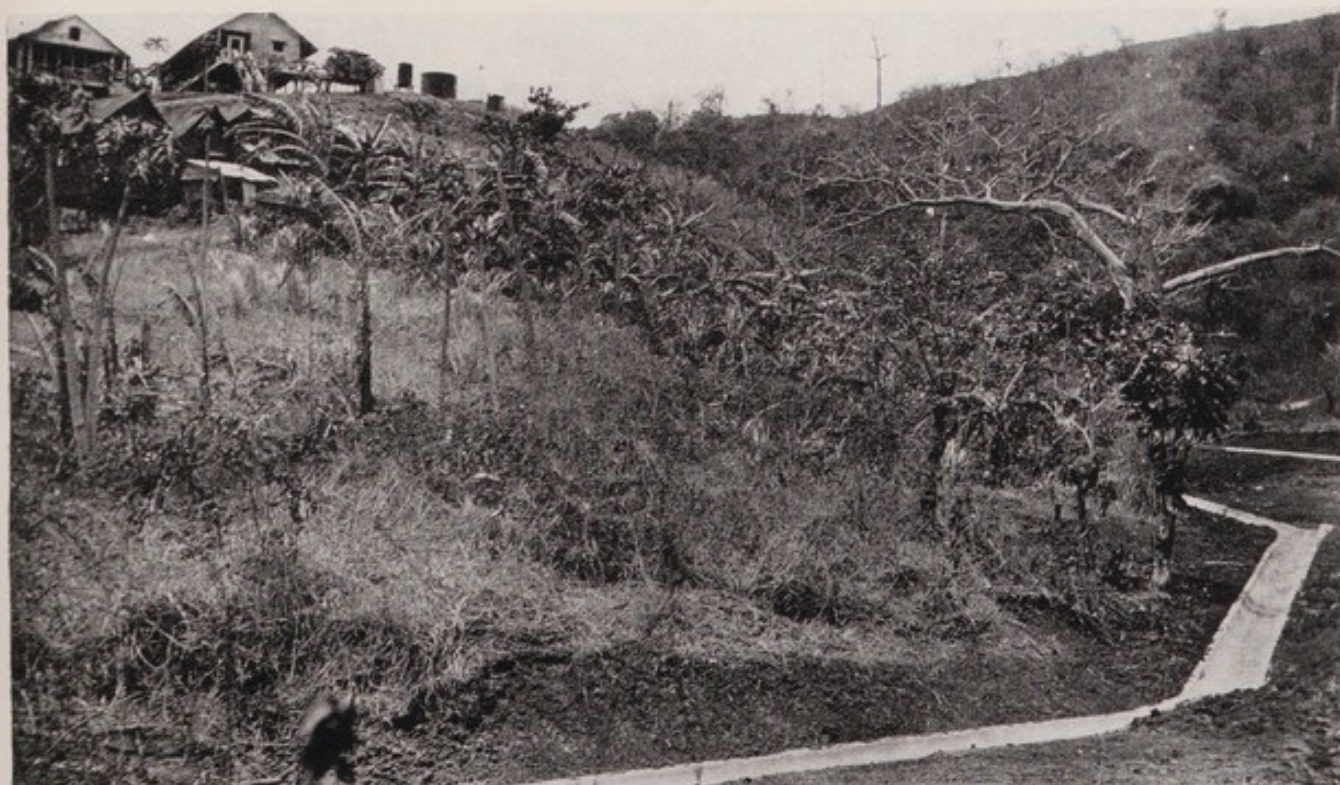
Concrete-lined ditch at Balboa
