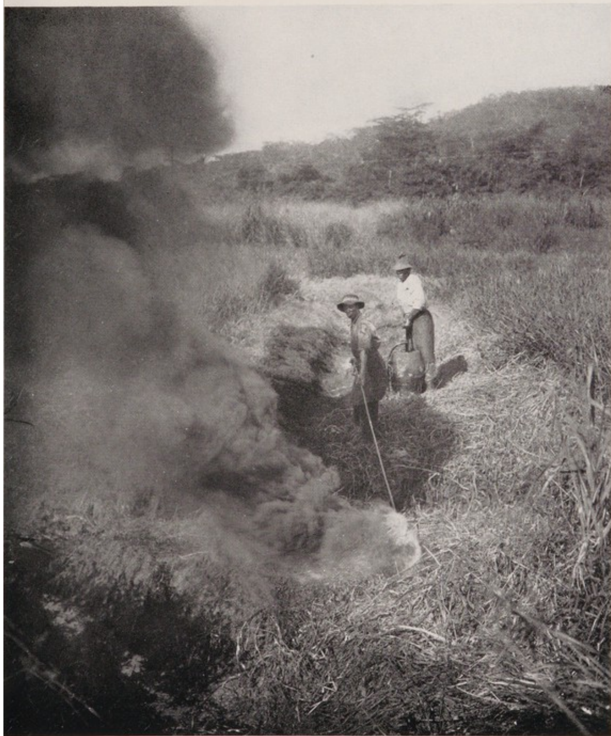
Burning grass from side of ditch; crude oil used as fuel
