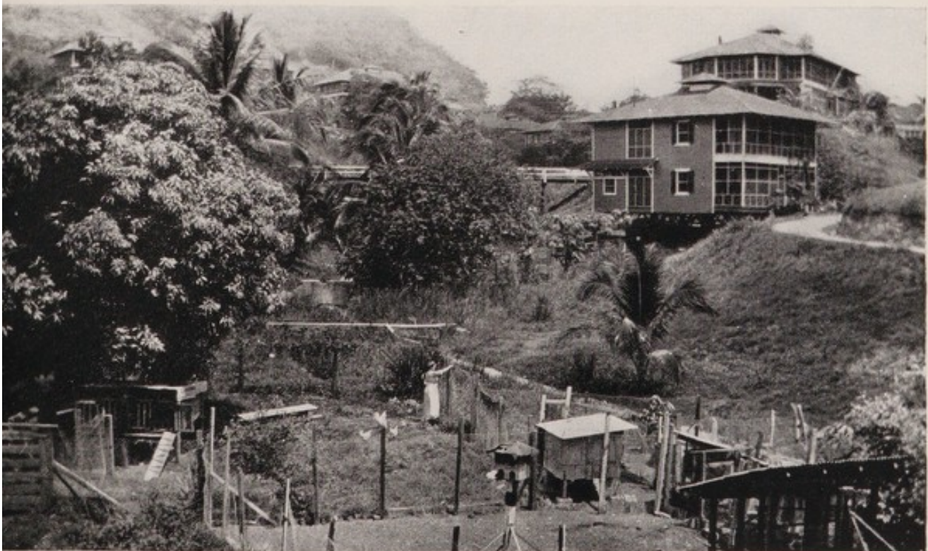
Screened verandas: Ancon
