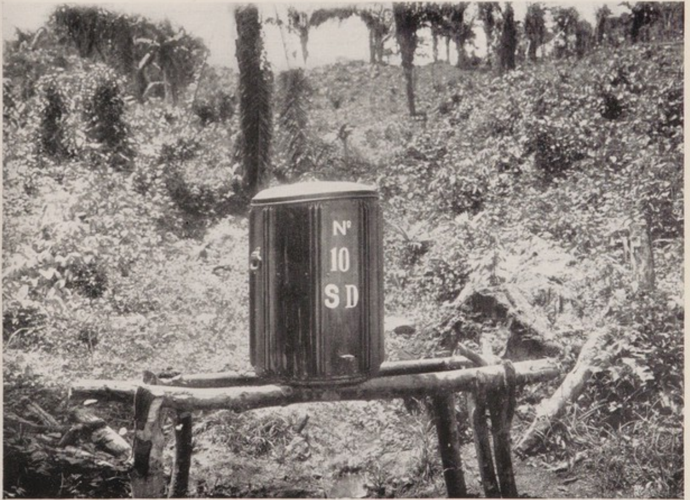
Oil drip applied to hillside stream
