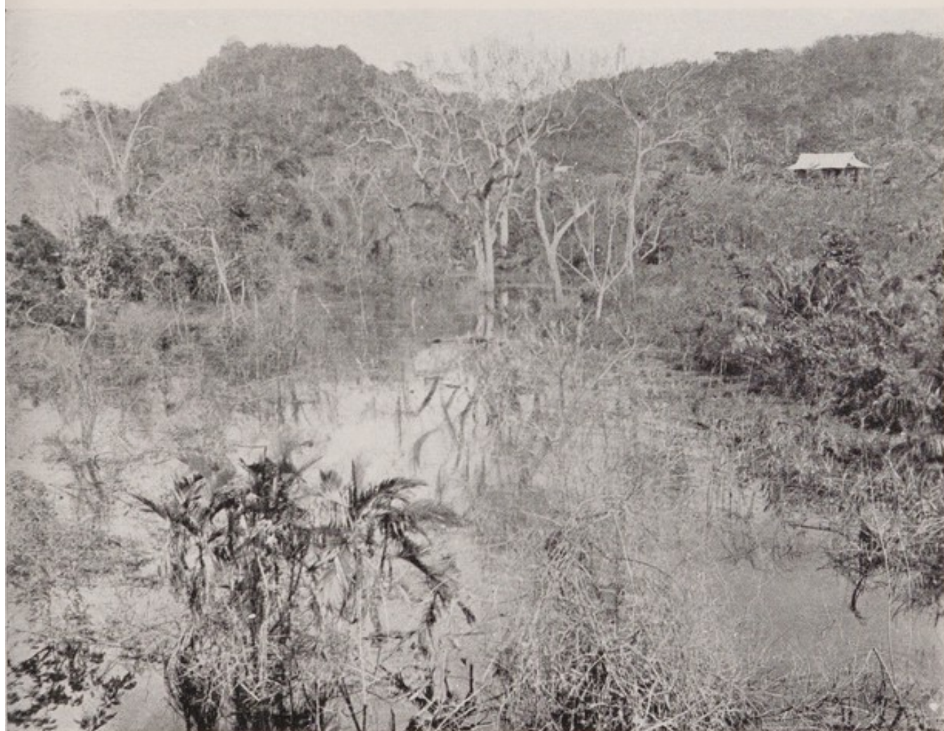
Blocked watercourse changed into an Anopheles breeding-place
