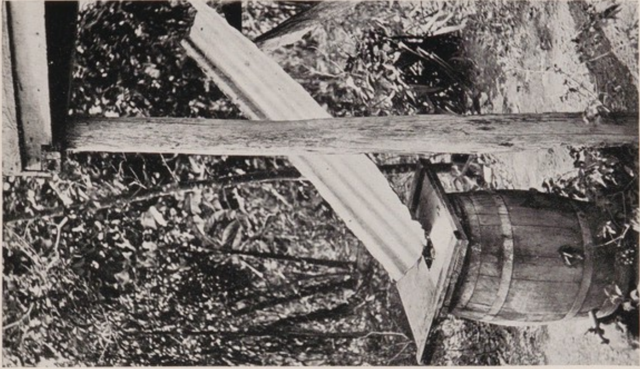
Mosquito-proof water-barrel
