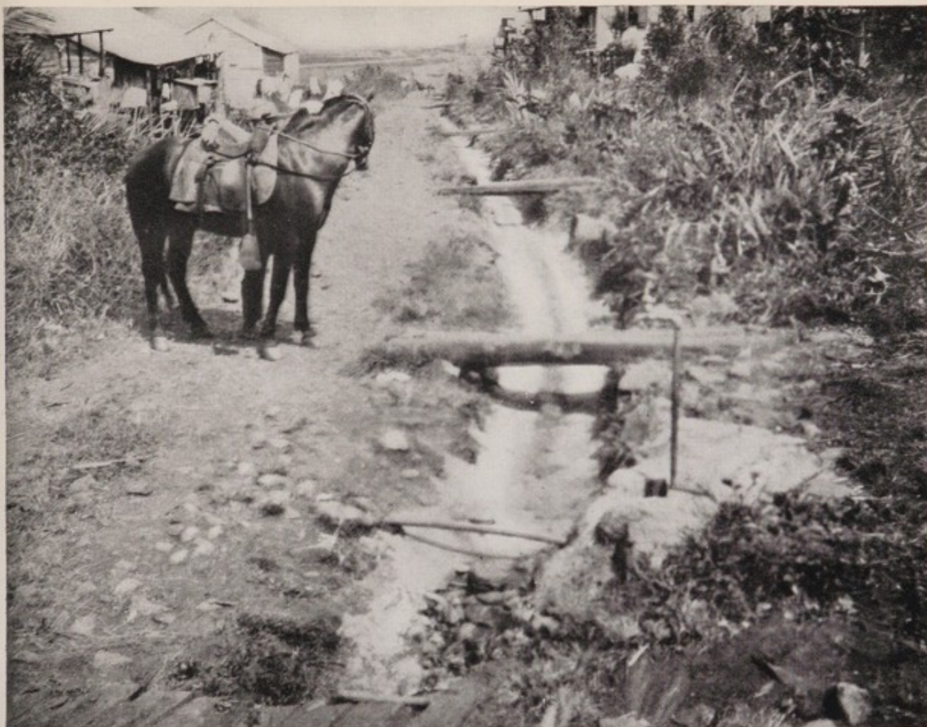
Concrete ditch lining
