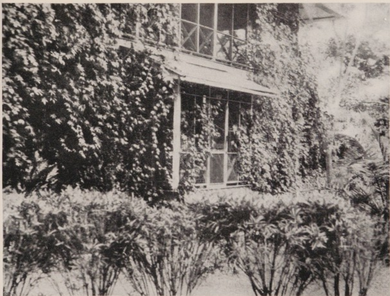
A short length of eave trough used over a doorway
