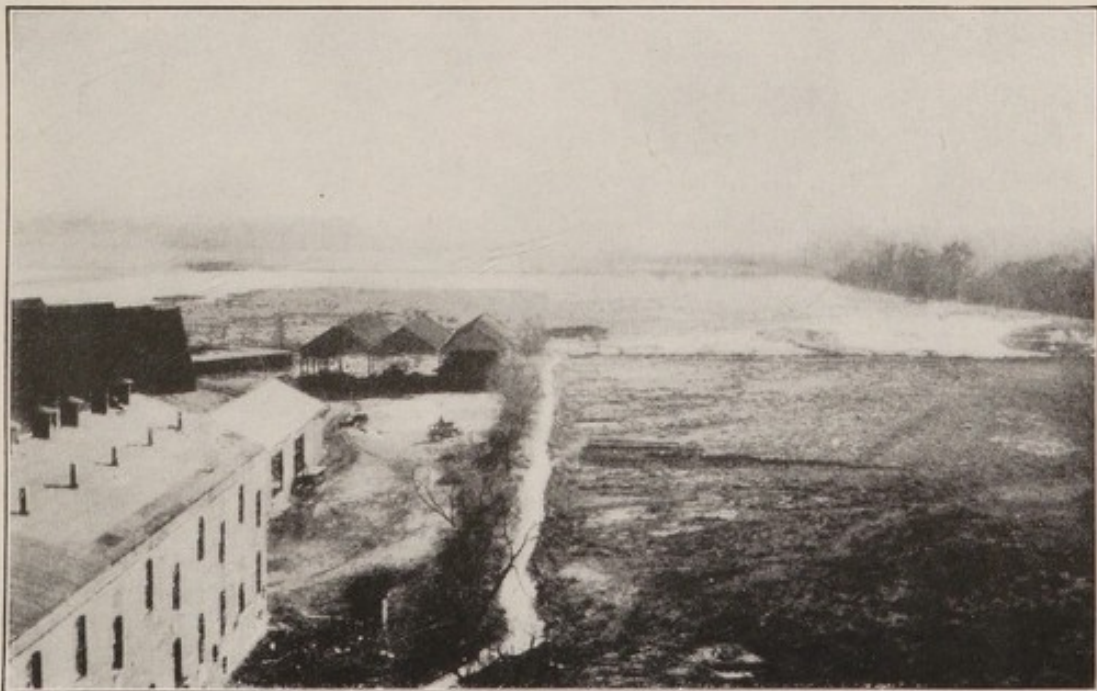
Fig. 2.—Effluent ditch and settling ponds.
