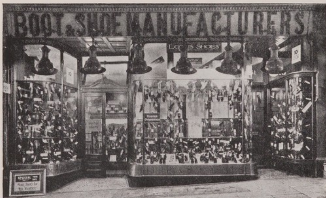
FIG. 174.—Window lighting by gas lamps, screened on the side facing the roadway.
