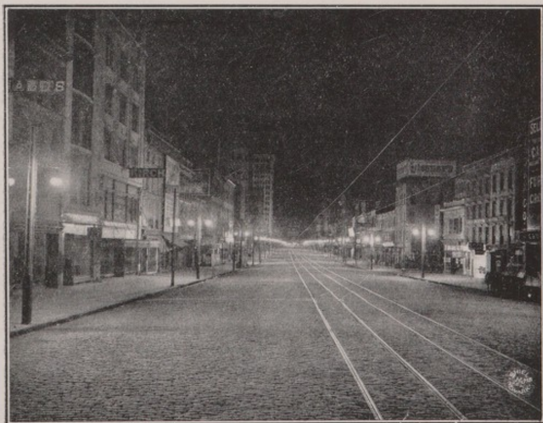
FIG. 194.—Very powerful pavement lighting by 10-amp. Excello are lamps, two on a post, only 16 feet above the ground and 50 to 75 feet apart.
