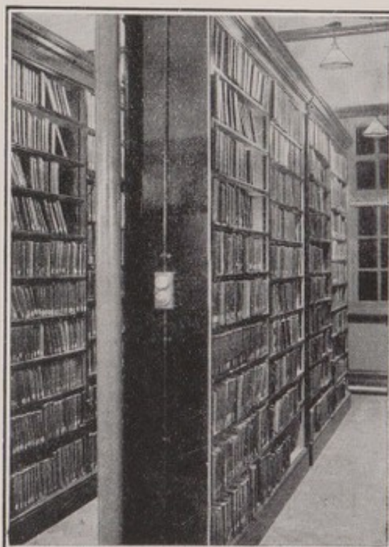
FIG. 156.—Rack lights by central tungsten lamps and Holophane reflectors (Enfield Public Library).
