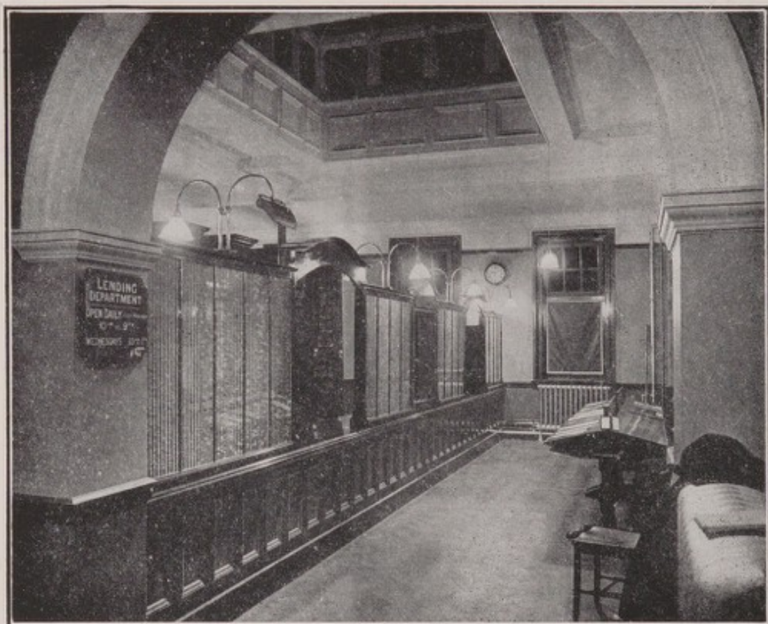
FIG. 157.—Enfield Lending Library, general illumination and local illumination of vertical registers by tungsten lamps and Holophane reflectors.
