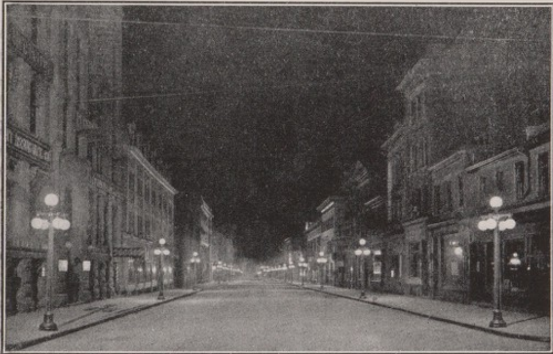
FIG. 186.—A street in Toronto lighted by clusters of tungsten lamps in Alba glass globes.
