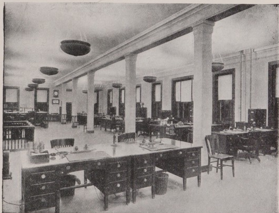
FIG. 126.—Indirect lighting in an office (B.T.H. "eye-rest" system).
