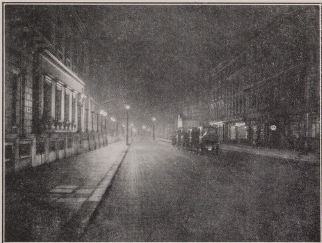
FIG. 182.—Lighting of Pall Mall, London, by high-pressure gas lamps “staggered” on either side of roadway.
