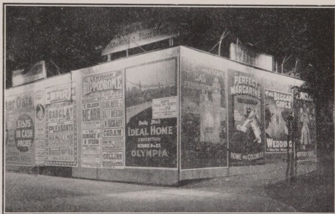
FIG. 196.—A series of posters in the district of the South Metropolitan Gas Co., London, illuminated by gas lamps with special opaque reflectors, distributing the illumination evenly over the surface.
