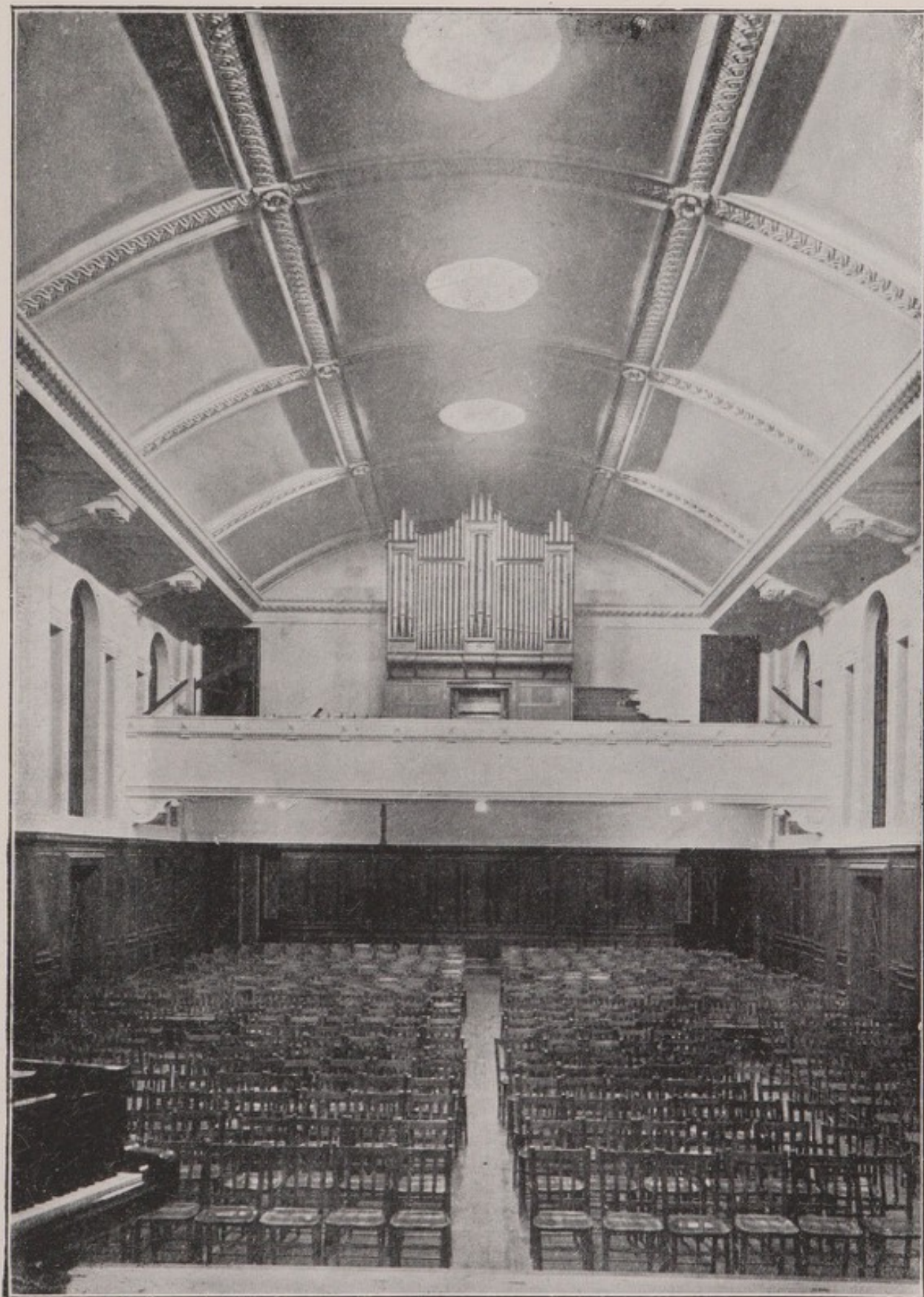
FIG. 167.—Assembly hall lighted by four "Nonpareil" sun-burners," consuming roughly one-ninth of a cubic foot of gas per square foot of floor area, the illumination produced being 8 foot-candles.
