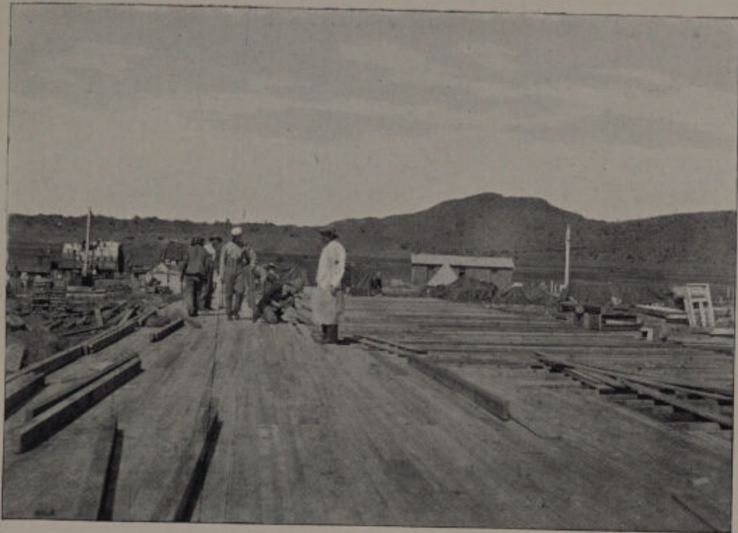
LAYING FLOOR OF BLOCK.
