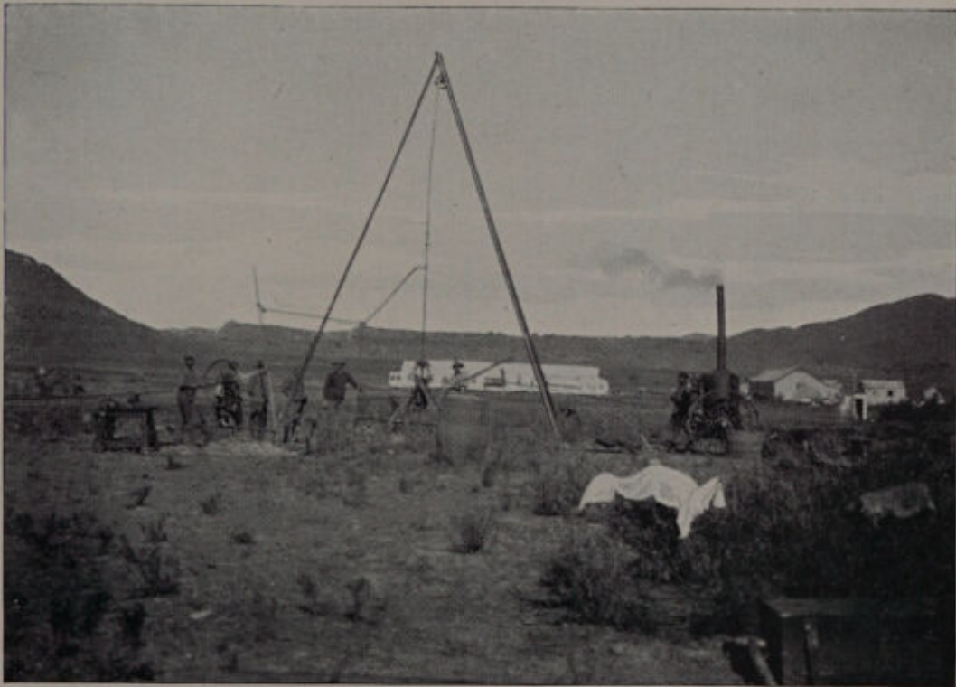
BORING FOR WATER.
