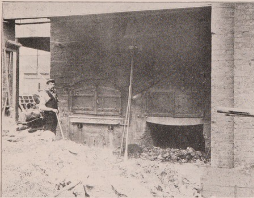
FIG. 1. THE FIRST TWO DESTRUCTOR CELLS ERECTED AT WATER STREET DEPÔT, MANCHESTER, IN 1876.
