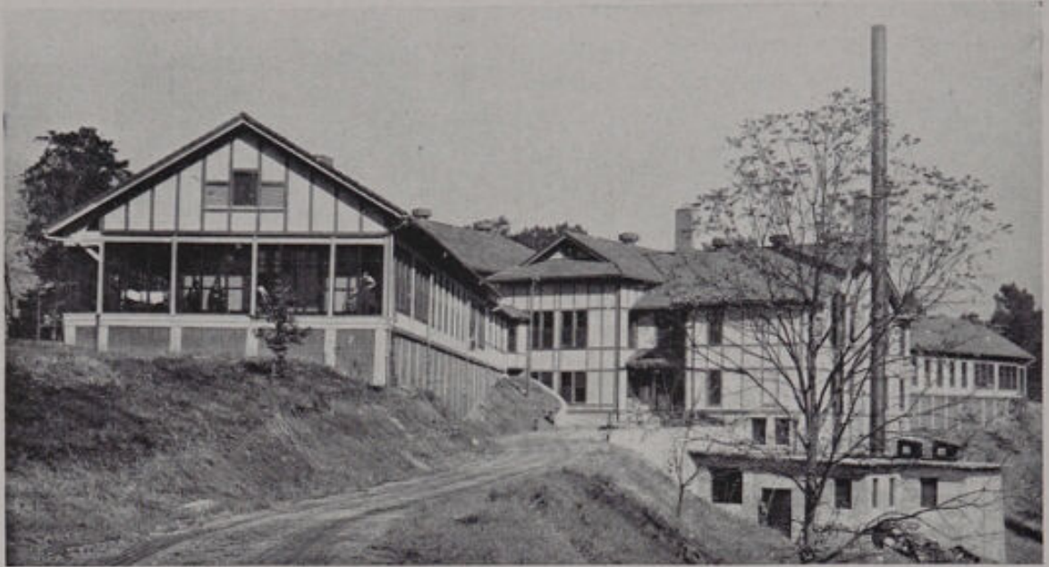
No. 18.—Waverly Hill Sanatorium, Waverly Hill, Ky. J. J. GAFFNEY, ARCHITECT. VIEW FROM THE REAR SHOWING A METHOD OF USING THE TOP AND SIDE OF A HILL IN ORDER TO OBTAIN A POSITION BELOW THE BUILDINGS FOR THE POWER PLANT. (See illustration 5 for further description of this institution.)
