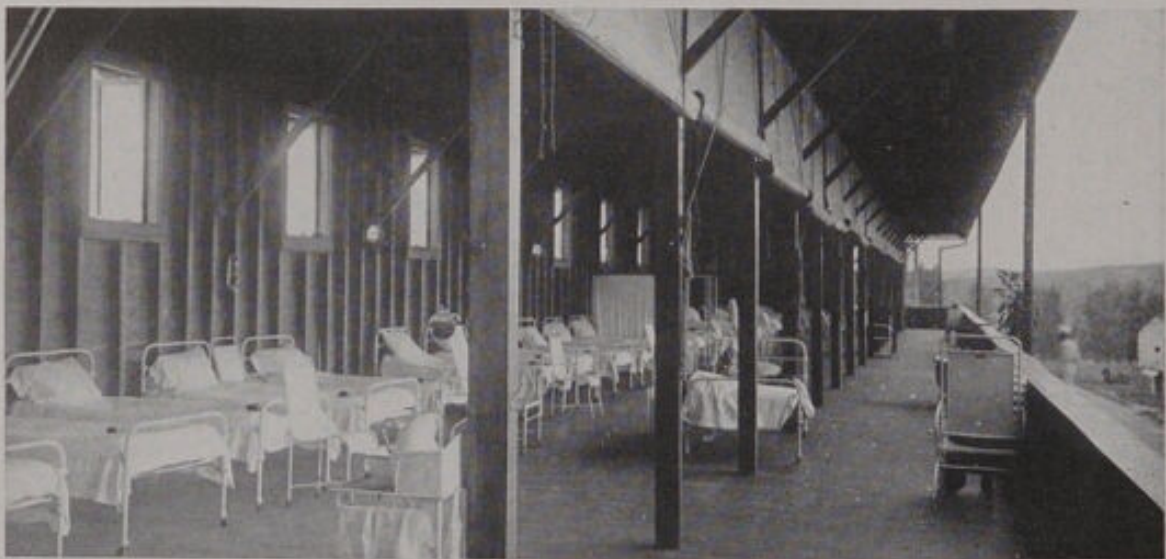
No. 71.—Virginia State Farm, Richmond, Va. VIEW OF OPEN PORCH ILLUSTRATING MANNER OF PROTECTING PORCHES BY CANVAS CURTAINS PLACED BETWEEN PILLARS, A FEW FEET BACK FROM THE LINE OF THE ROOF PROJECTION.
