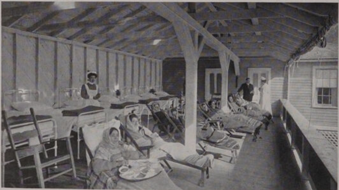
No. 69.—Catawba Sanatorium, Catawba, Va. DESIGNED BY DR. ENNION G. WILLIAMS. VIEW OF AN OPEN PORCH ILLUSTRATING A METHOD OF CONSTRUCTION WITHOUT INTERIOR FINISH, AND A MANNER OF PROTECTING PORCHES BY CANVAS CURTAINS UNDER THE EDGE OF THE ROOF PROJECTION. (See illustrations 17, 30 and 80 for further description of this institution.)
