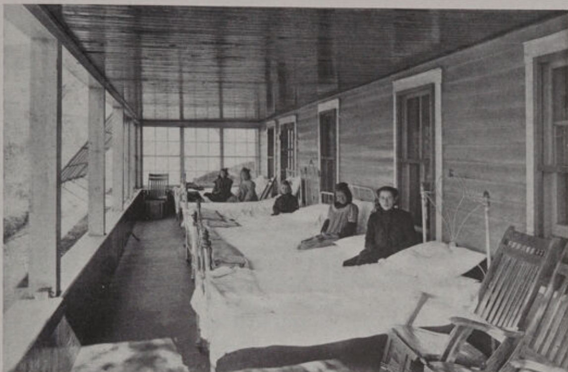
No. 72.—Loomis Sanatorium, Liberty, N. Y. VIEW OF CHAPMAN COTTAGE. SLEEPING PORCH; ILLUSTRATING METHOD OF CONSTRUCTION AND INTERIOR FINISH, USING NARROW FLOOR BOARDS FOR SEALING. (See illustrations 1, 73, 91 and 108 for further descriptions of this institution.)
