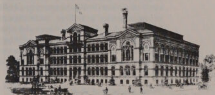
Library building on the mall, opened in 1887.
