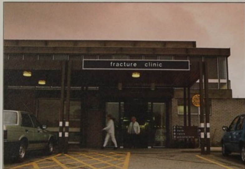
The new entrance to the fracture clinic.
