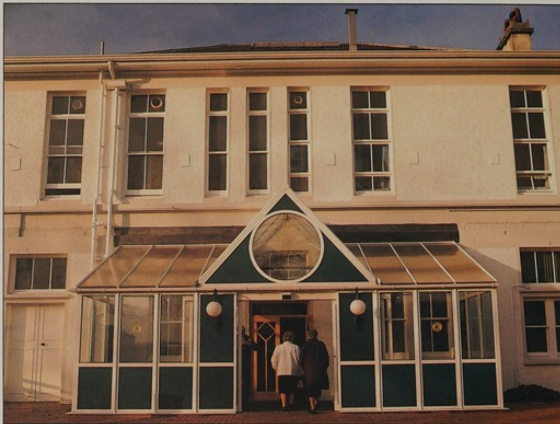
The conservatory replaced the run-down, narrow entrance below.
