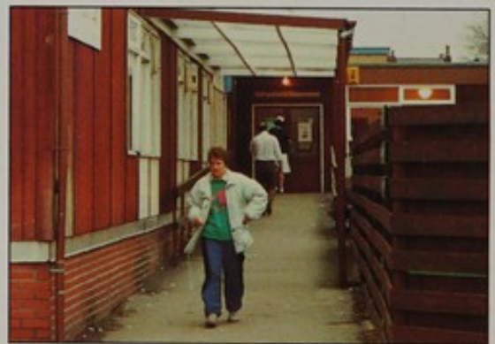
The old main entrance.
