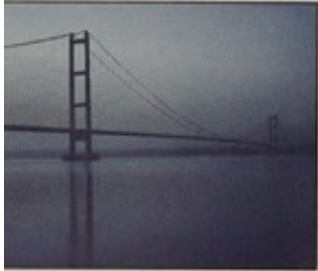
The Humber Bridge.
