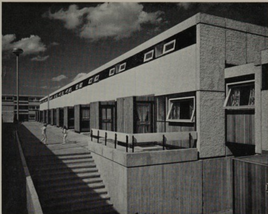
22 Storey-height timber cladding. The photograph shows use of storey-height timber cladding on the ground floor of 2B4P-type dwellings.
