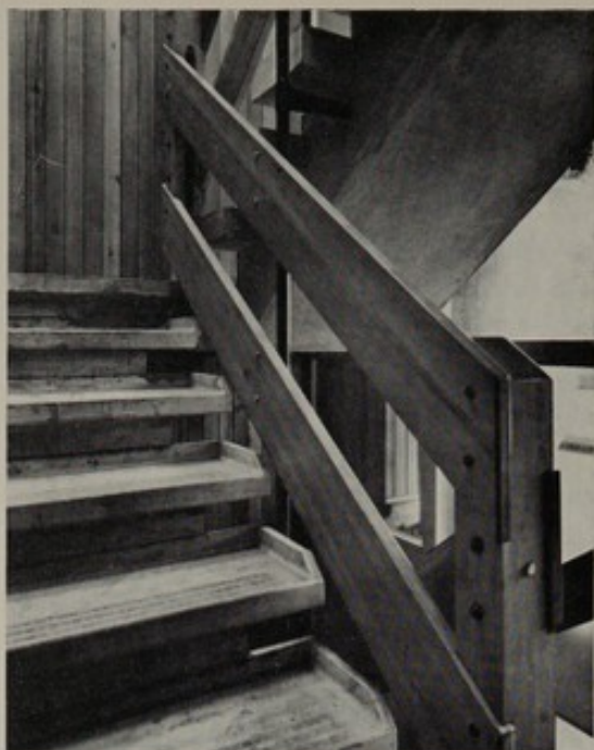
(a) Details of precast treads and timber handrail;
