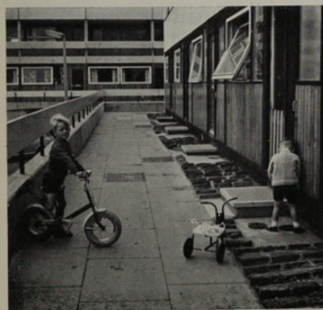
42 and 43 Two examples of barrier paving to stop passers-by approaching too close to the dwelling. Constructed of setts which formed the surface of the roads before redevelopment; the angled version (Figure 43) had the advantage of being more effective but had the disadvantage of holding dirt, cigarette ends, waste paper etc.
