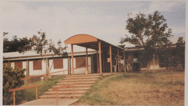
Isiolo Hospital, Kenya (Appendix 3A)
