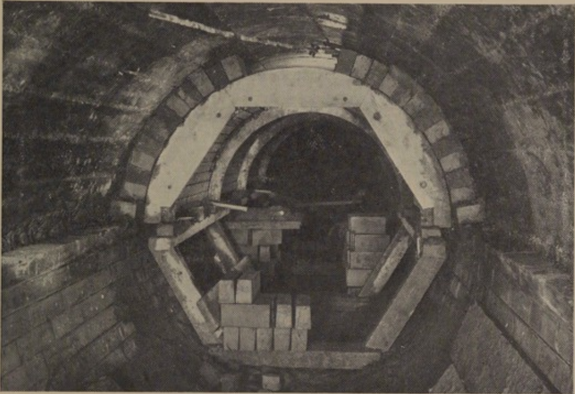
MAIN TRUNK SEWER—CATHERINE STREET TO PLASMARL (Brick lining under construction within completed concrete lining)
