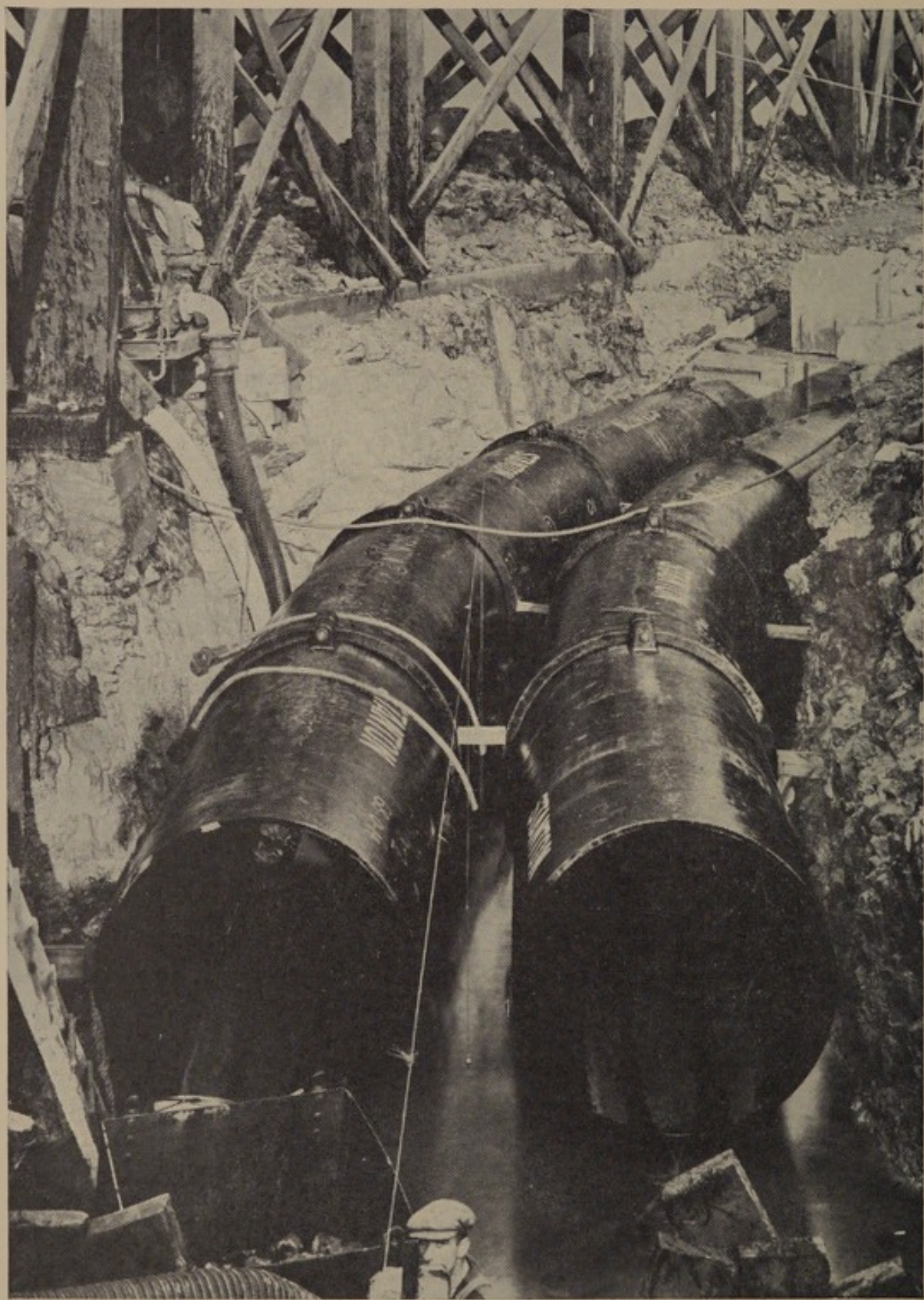
SEA OUTFALL—CAST IRON PIPES IN TRENCH
