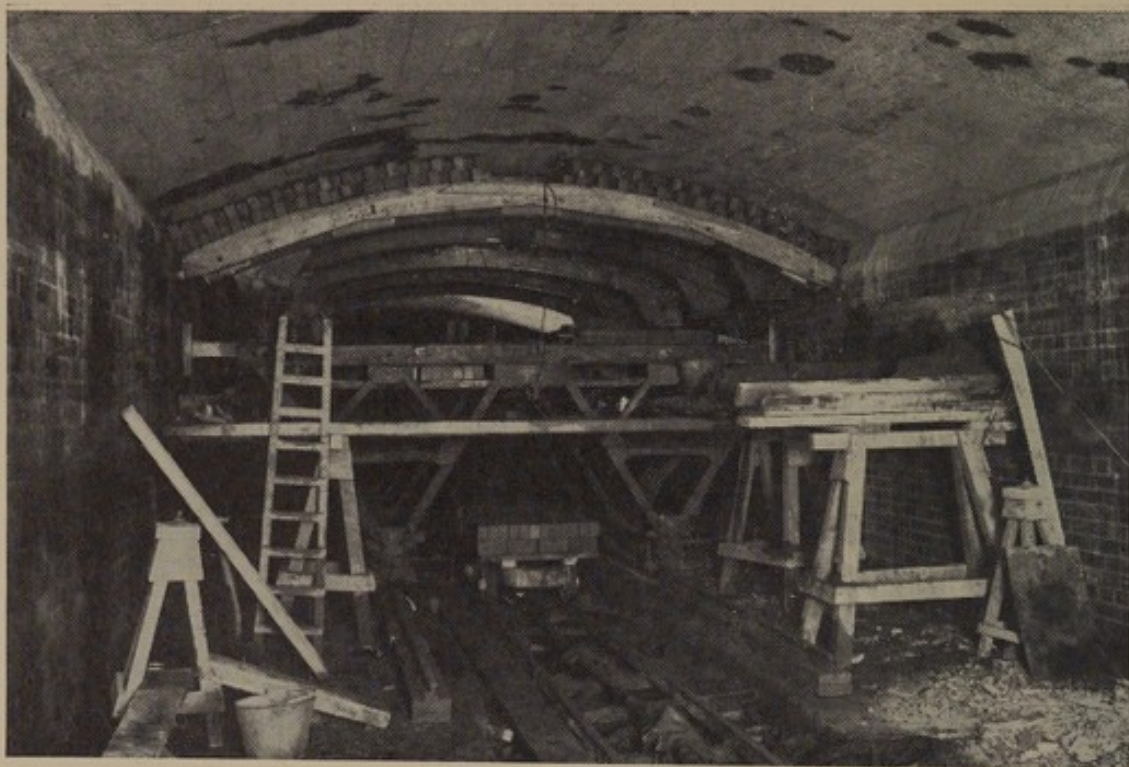
STORAGE TANKS (Concrete and brickwork lining under construction)
