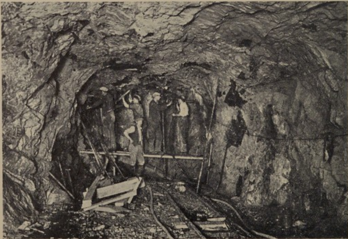
STORAGE TANKS—Drilling at face preparatory to blasting.
