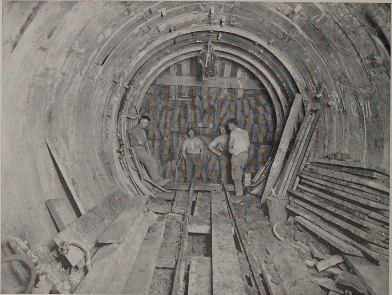
CONCRETE SEGMENT TUNNEL FOR 9-FEET DIAMETER SEWER.
