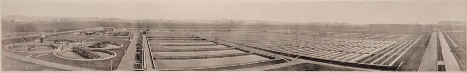
PRIMARY SEDIMENTATION TANKS
