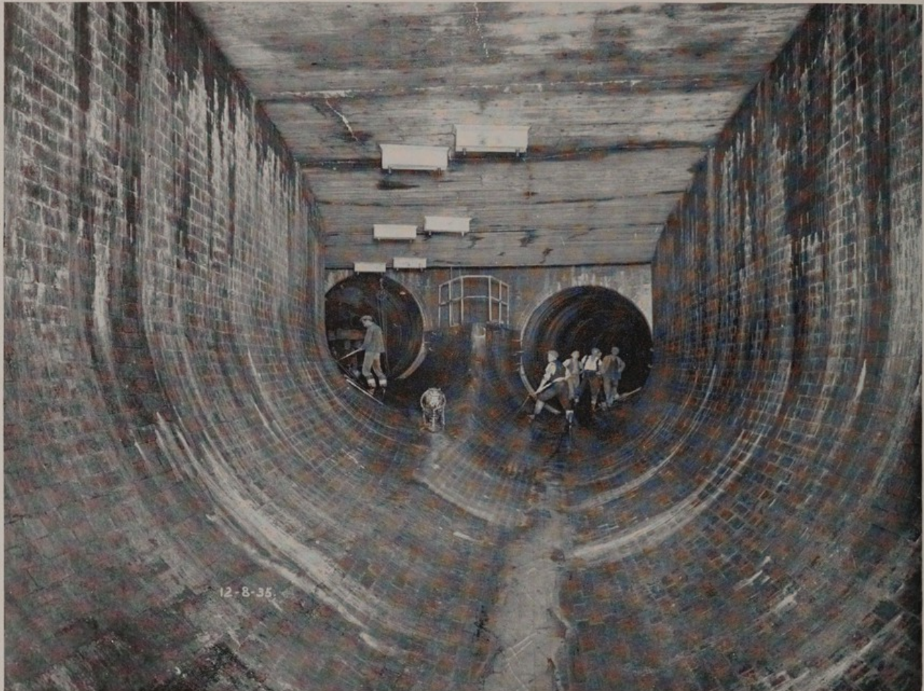
JUNCTION CHAMBER. 9-FEET, 10-FEET 9-INCHES AND 12-FEET 9-INCHES DIAMETER SEWERS.
