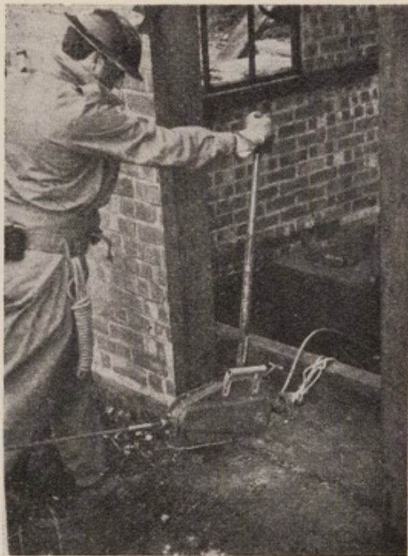
Fig. 107. Attached to base of concrete fence post
