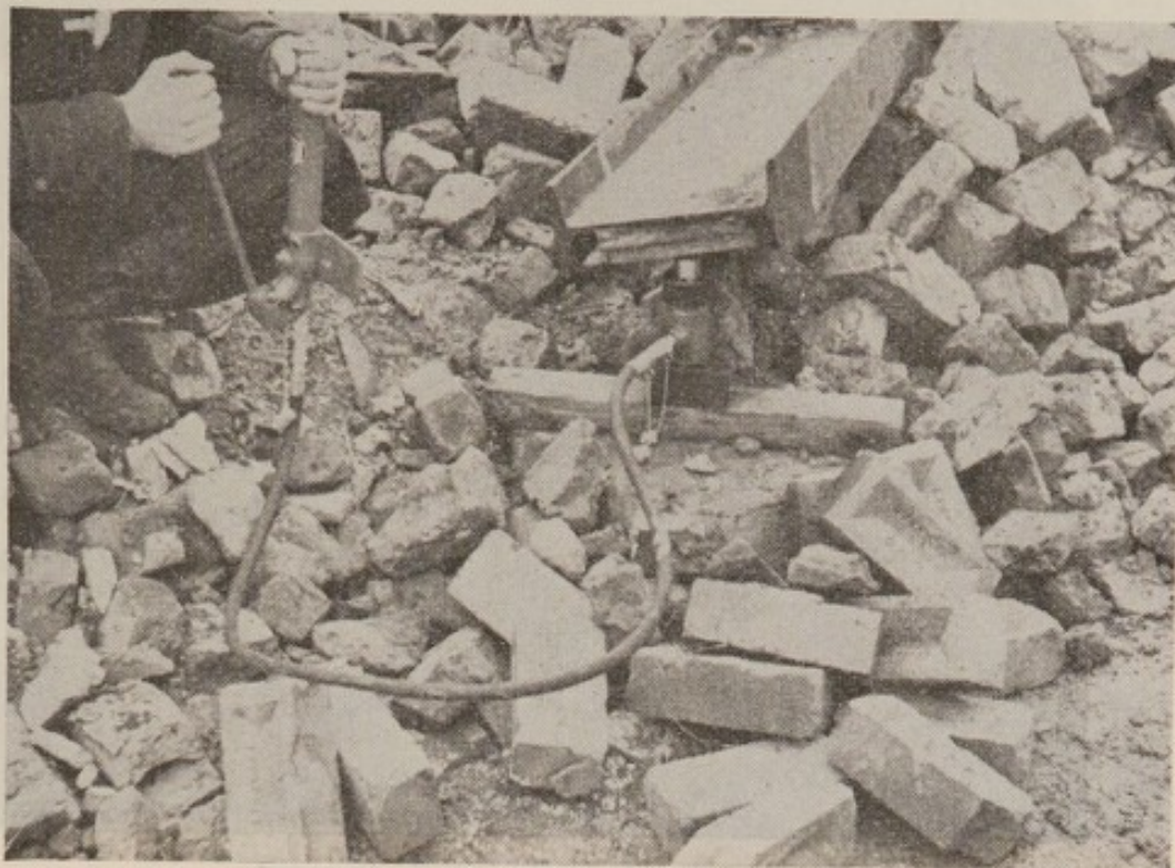
Fig. 117. A straight-forward lift by the ram
