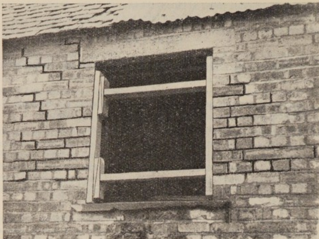
Fig. 69 (a). Strutting of window opening
