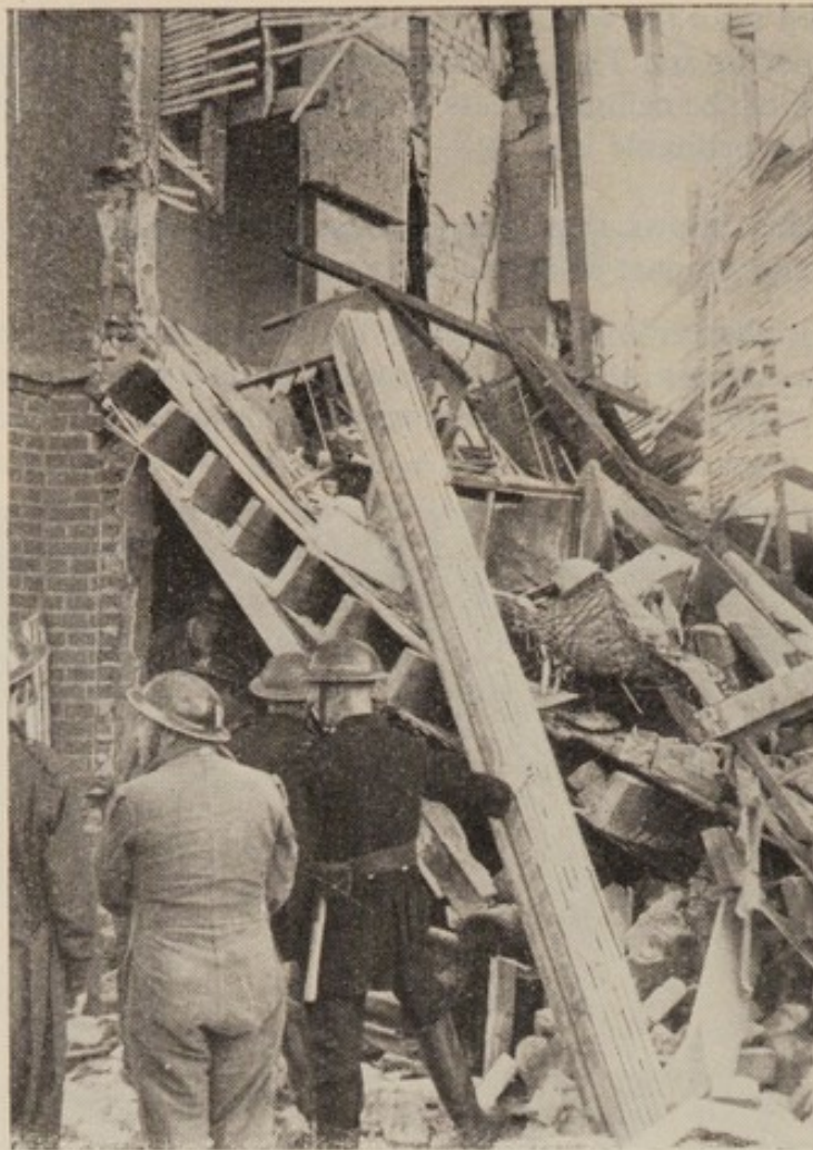
Fig. 79. Example of lean-to collapse (not in basement)
