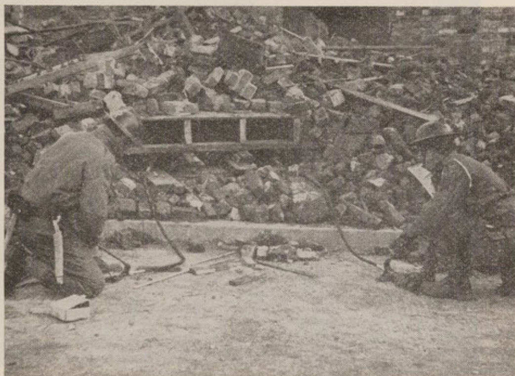
Fig. 121. Utilising both rams in unison
