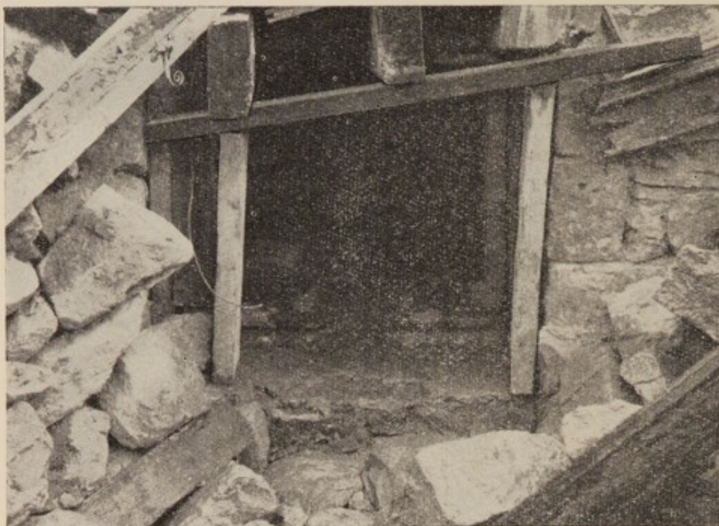
Fig. 71. Temporary strutting
