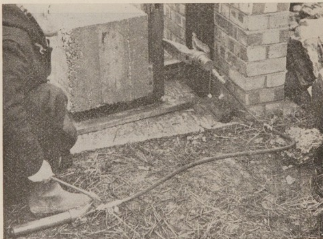
Fig. 122 (b). Another use of the alligator spreader
