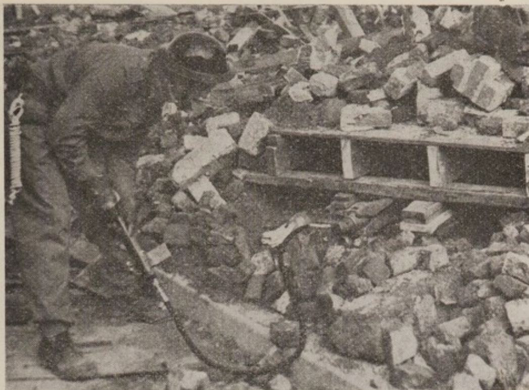
Fig. 120. Initial lift by the alligator spreader
