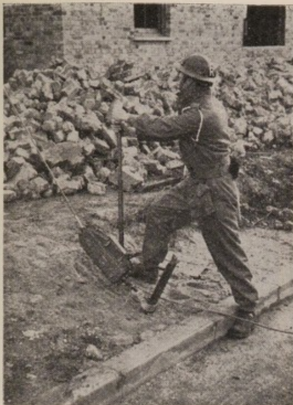
Fig. 105. Using a piece of debris steel as holdfast
