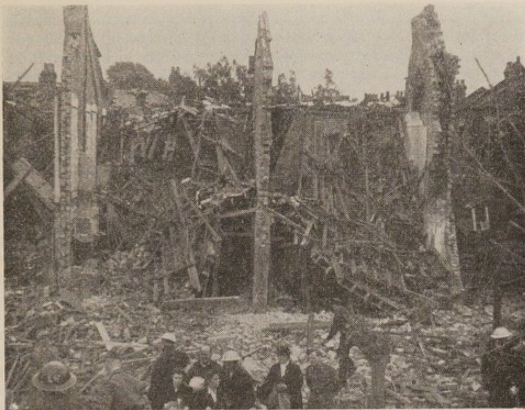
Fig. 9. Note how voids have been formed by the collapse of floors
