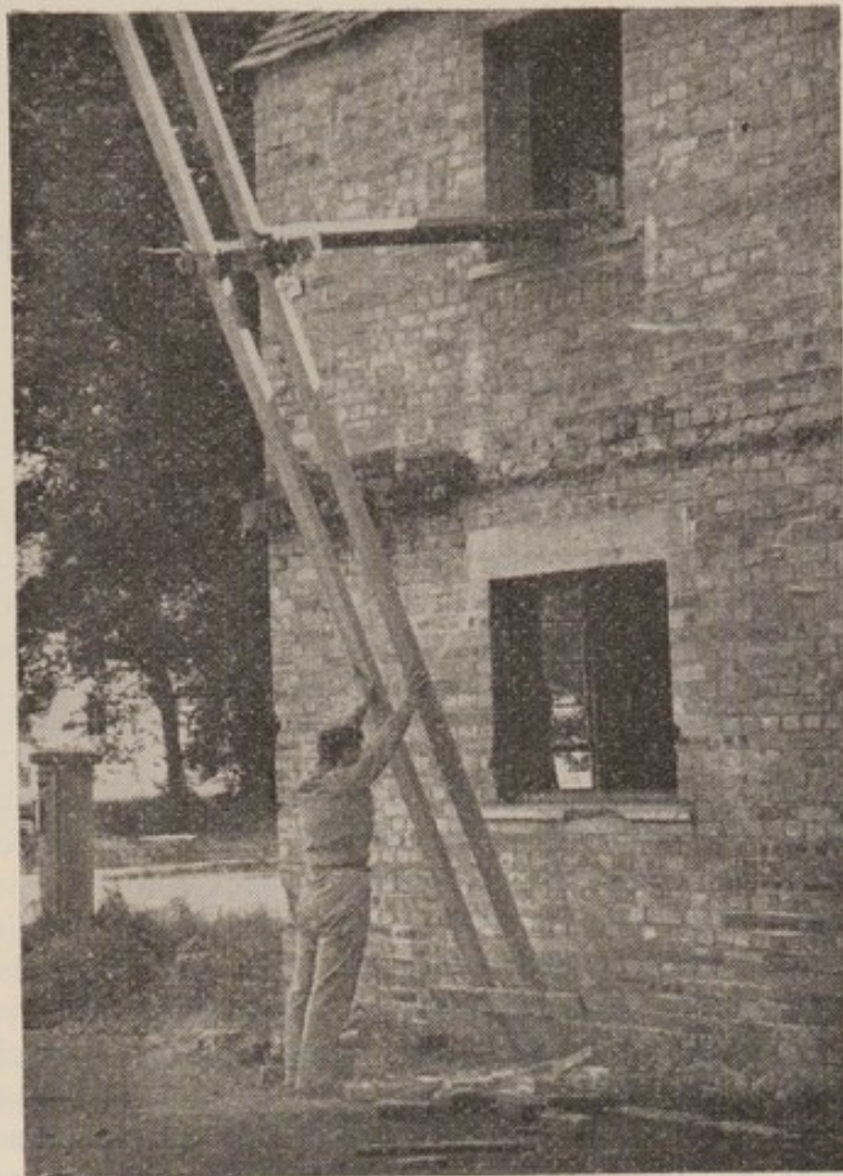
Fig. 99 (c). Another form of improvised ladder hinge
