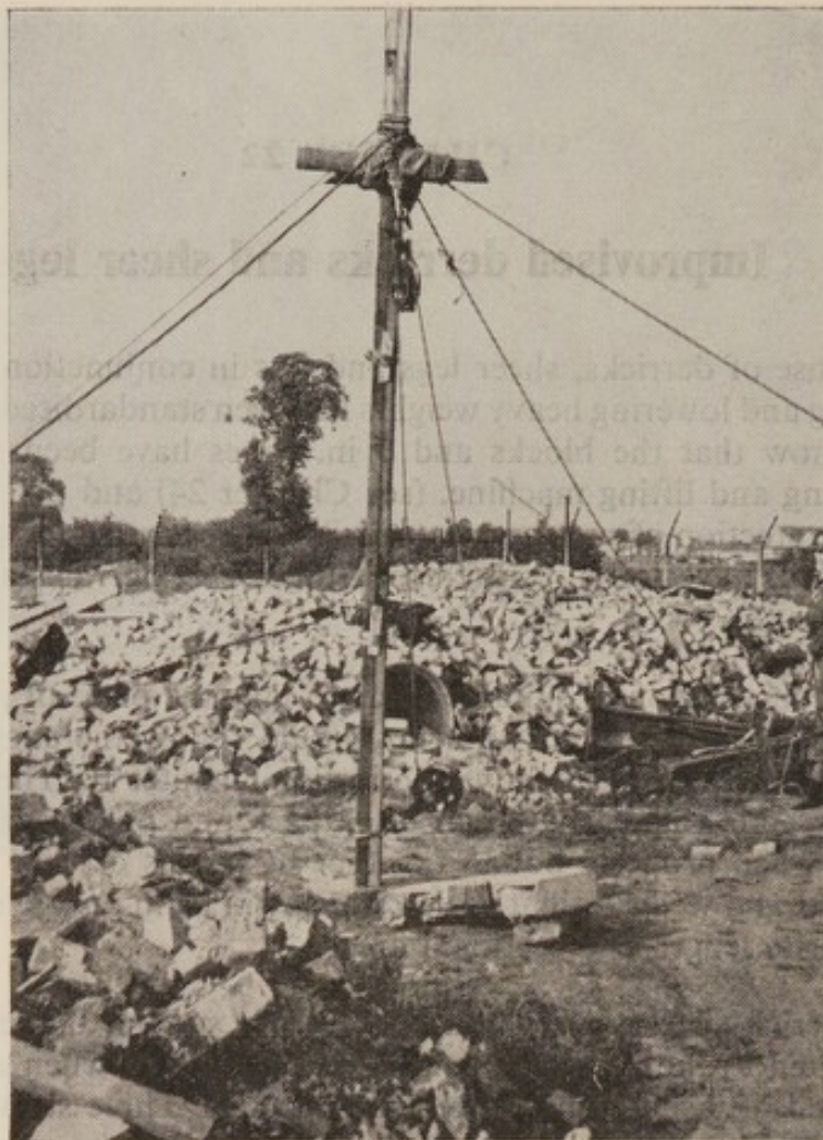
Fig. 90. An improvised derrick
