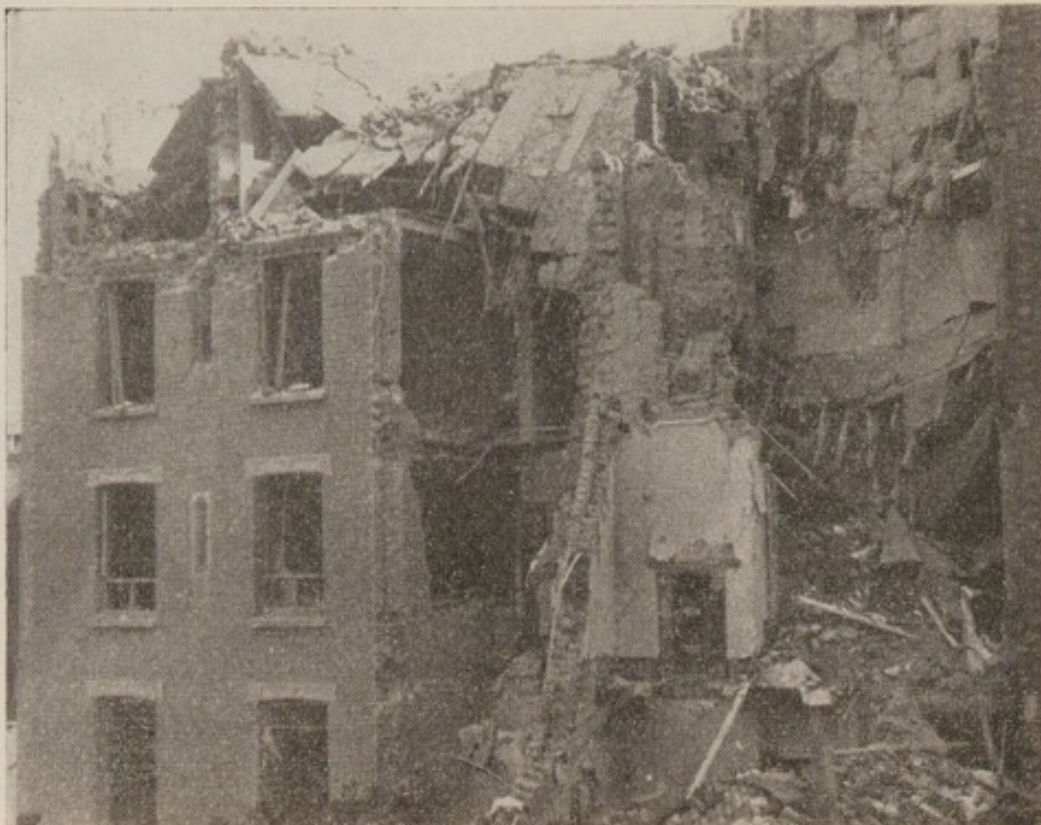
Fig. 7. Unframed building showing how walls support the floors (note collapsed concrete roof)
