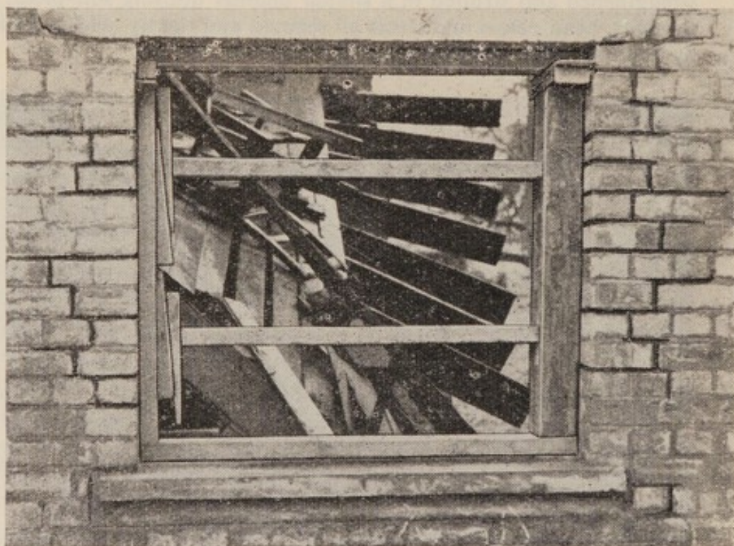
Fig. 69 (b). Strutting of window opening
