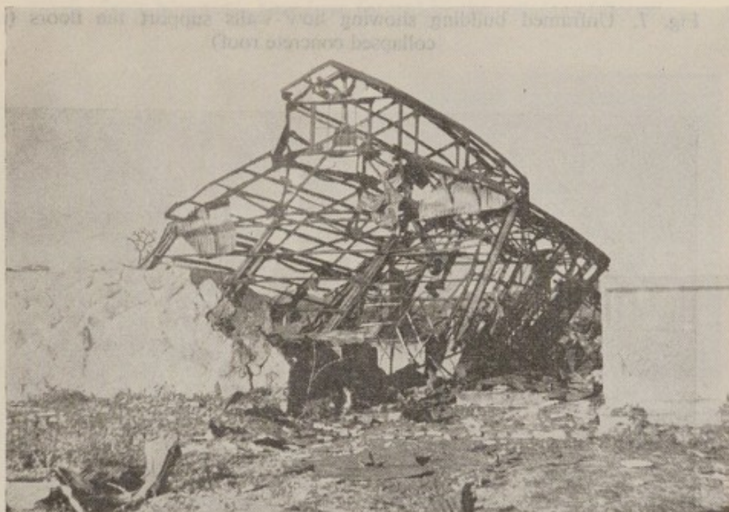
Fig. 6. Steel framed building distorted away from the explosion: Hiroshima, 1945
