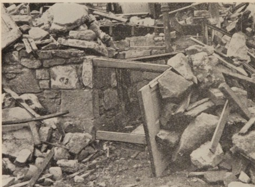
Fig. 72. Utilising an old door, strutted back from the remains of a stone wall, to hold up debris and form a crawlway for the extrication of casualties
