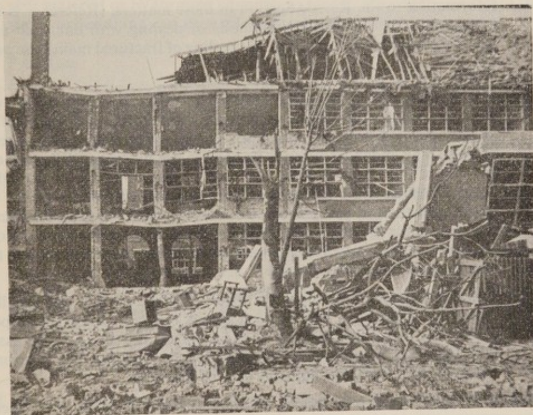
Fig. 10. Effects of blast damage on a framed building
