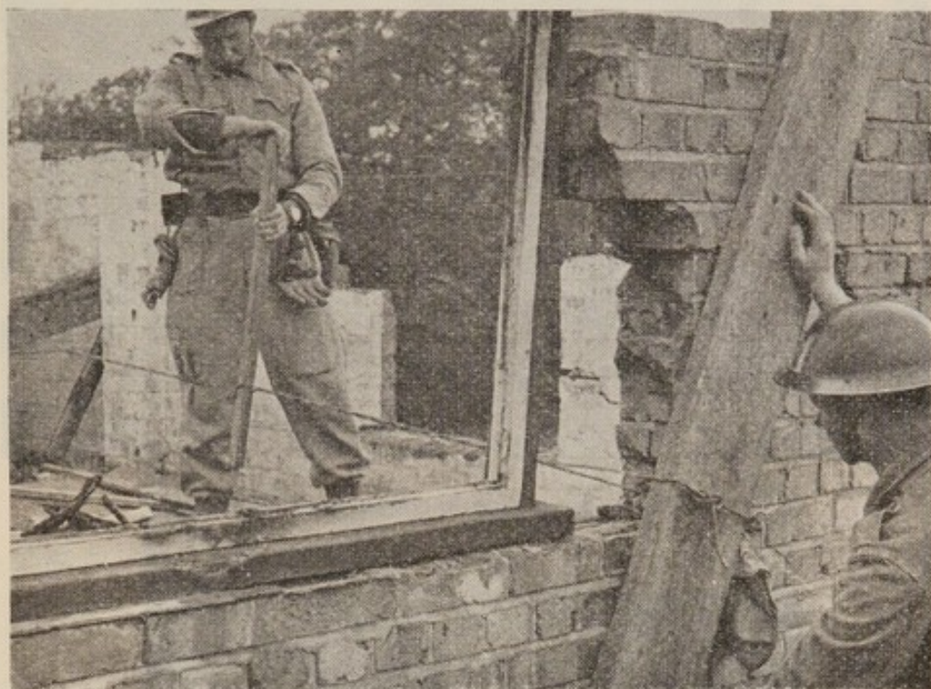
Fig. 22. Horizontal support of unsafe wall
