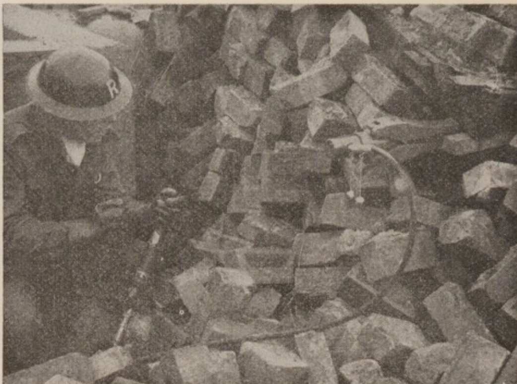
Fig. 122 (a). Another use of the alligator spreader
