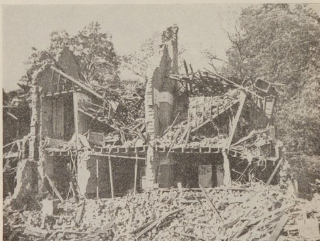
Fig. 8. Effect of blast damage on unframed buildings
