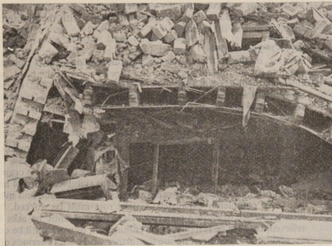
Fig. 83. Debris crawlway
