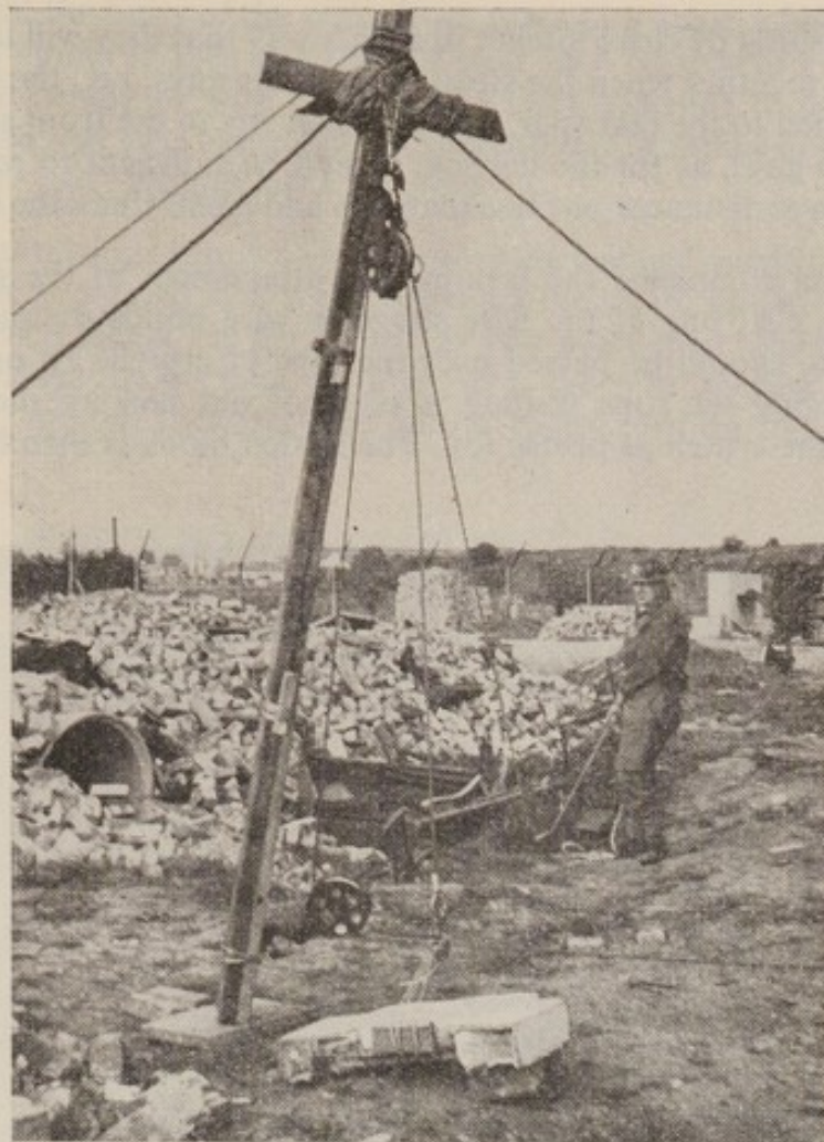
Fig. 92. Luffing a derrick
