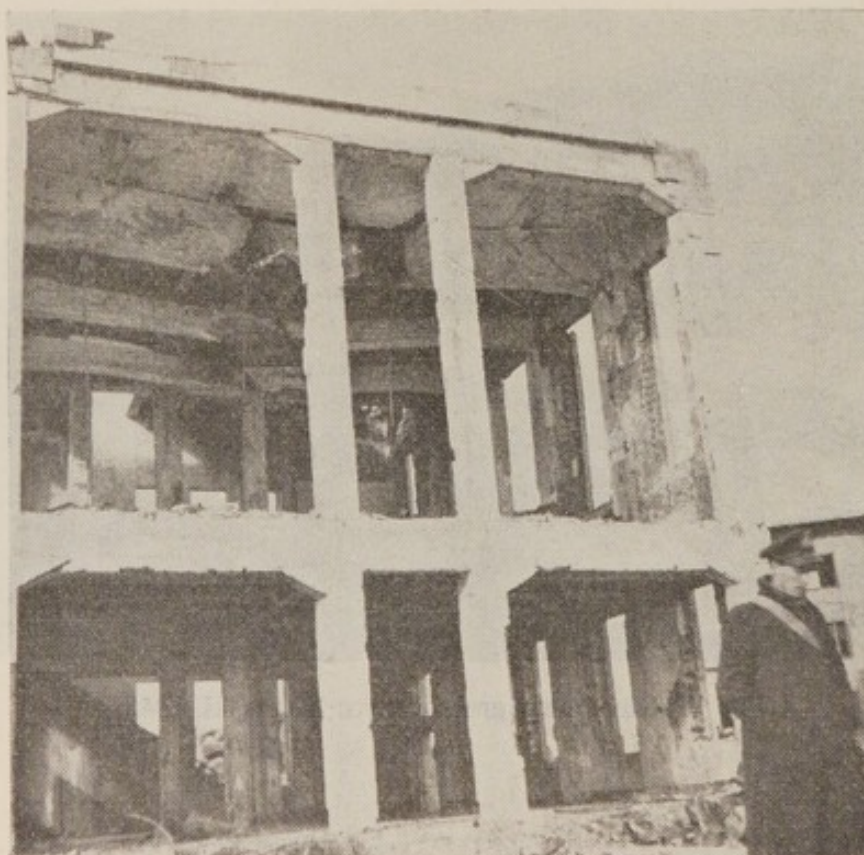
Fig. 4. Roofs are dished in by downward blast: Nagasaki, 1945
