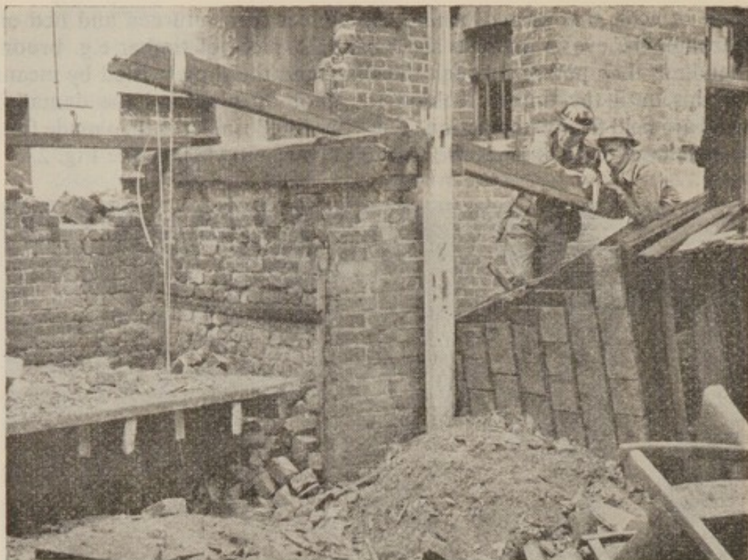
Fig. 23. Wire bond sling in conjunction with a spar
