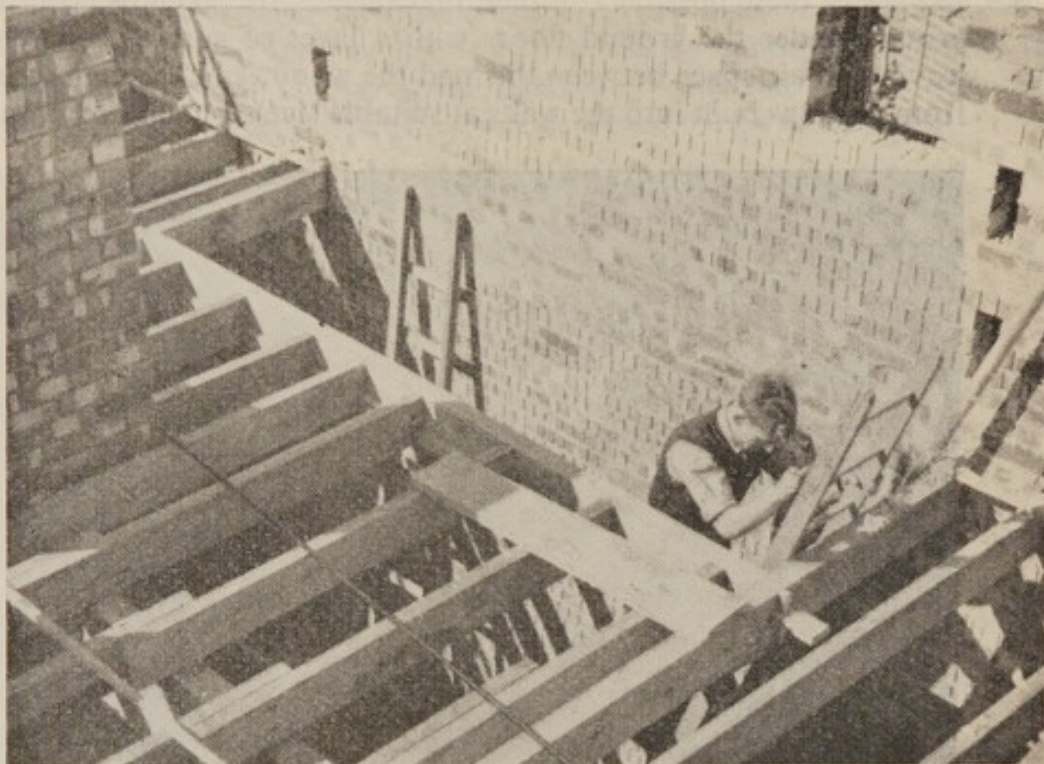
Fig. 14. Upper floor joists trimmed for staircase
