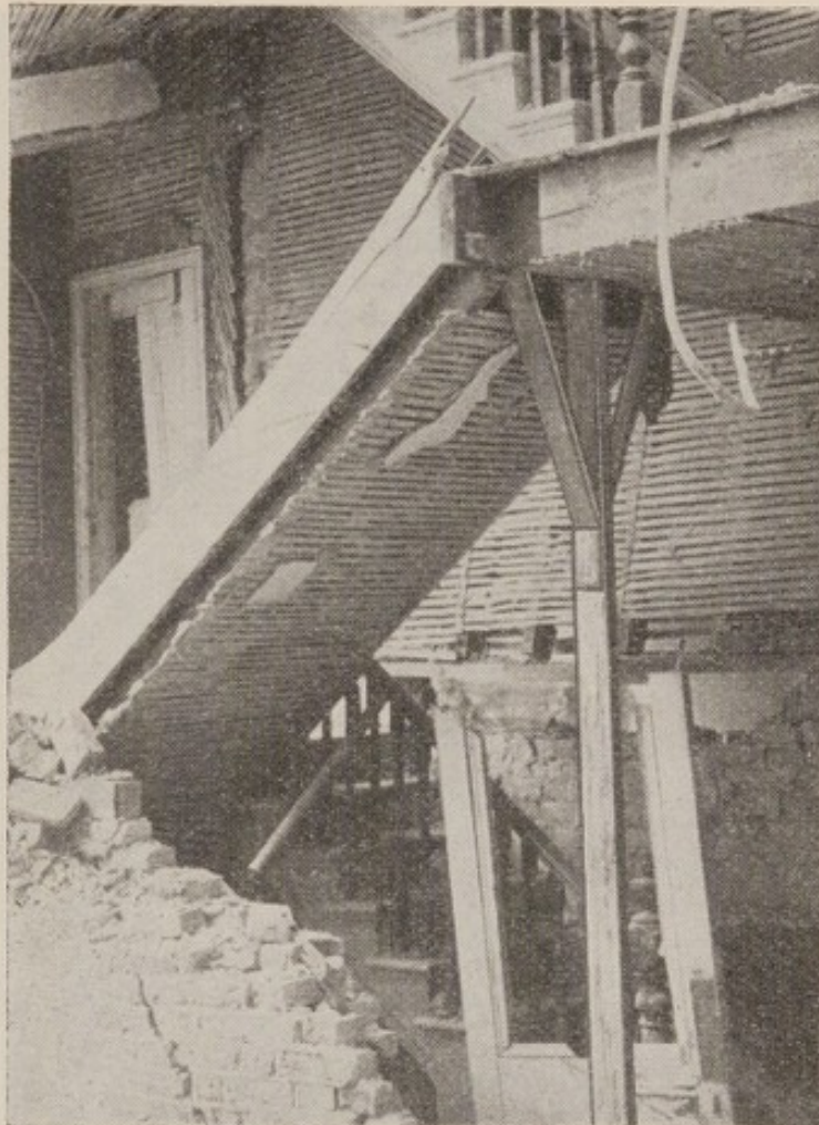
Fig. 125. Temporary shoring showing propping
