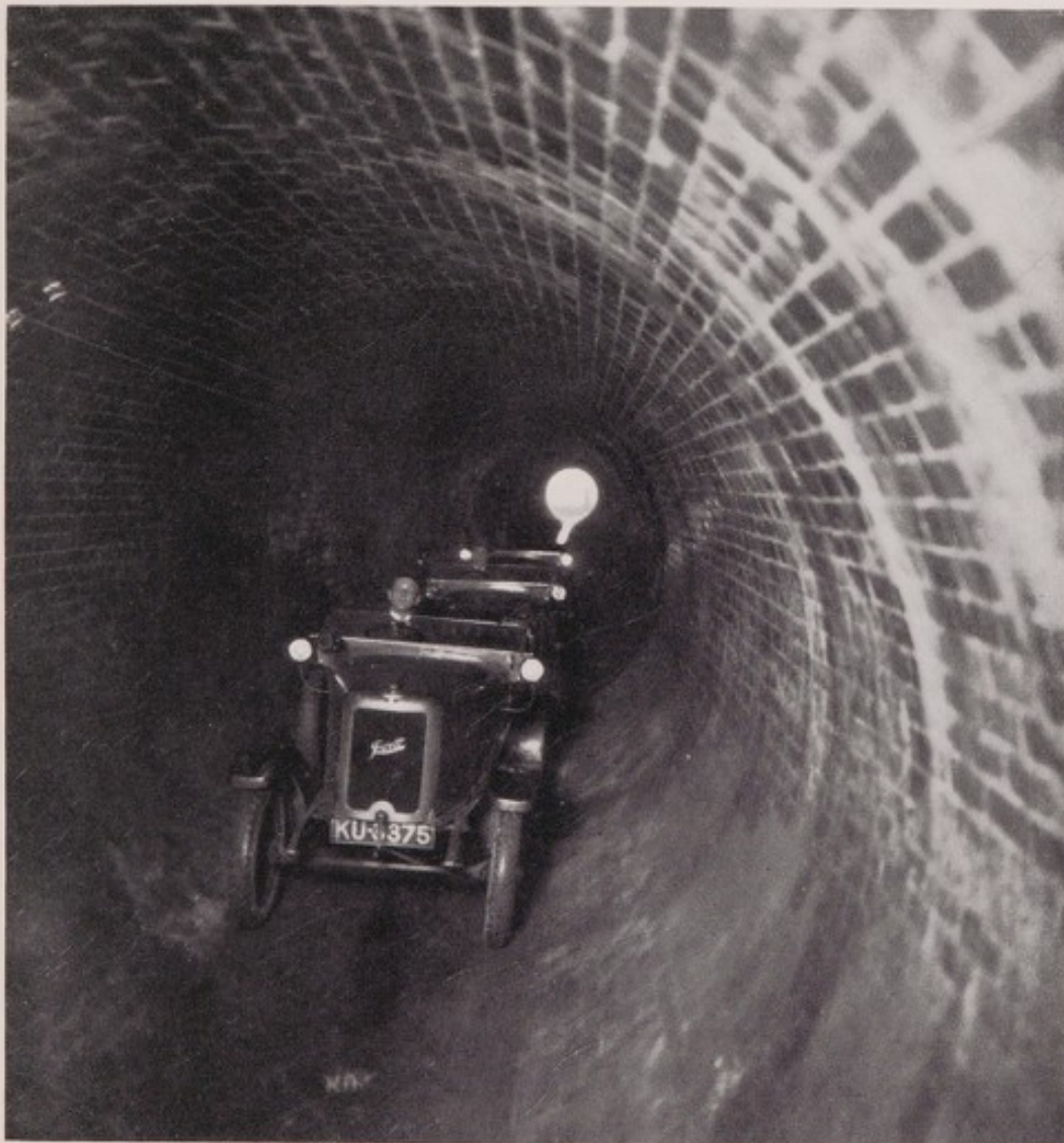
MOTOR CARS IN FINISHED TUNNEL SEWER.
