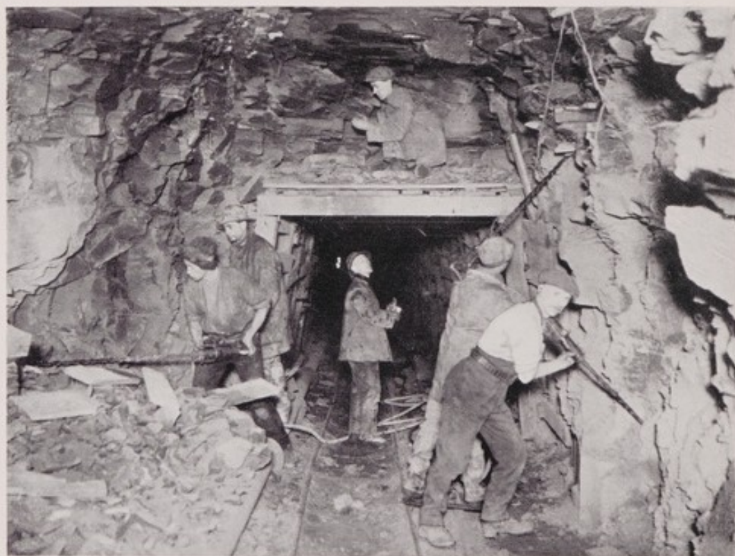
TUNNEL SEWER—ADVANCE HEADING.
