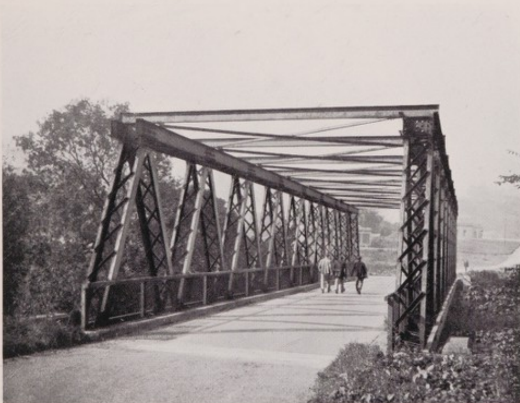
ROAD BRIDGE ACROSS THE RIVER AIRE.
