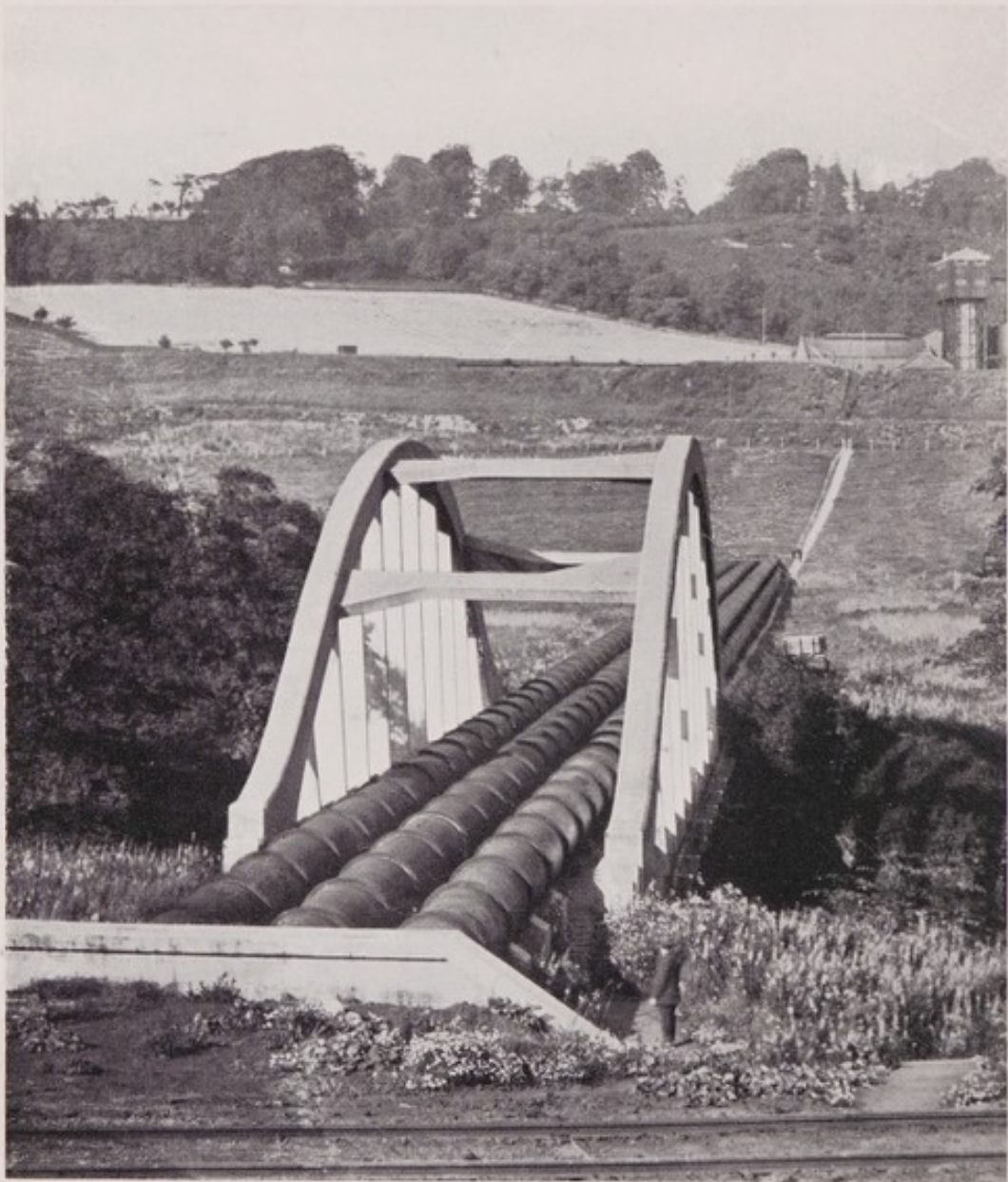
REINFORCED CONCRETE BRIDGE CARRYING SYPHON PIPE LINES.
