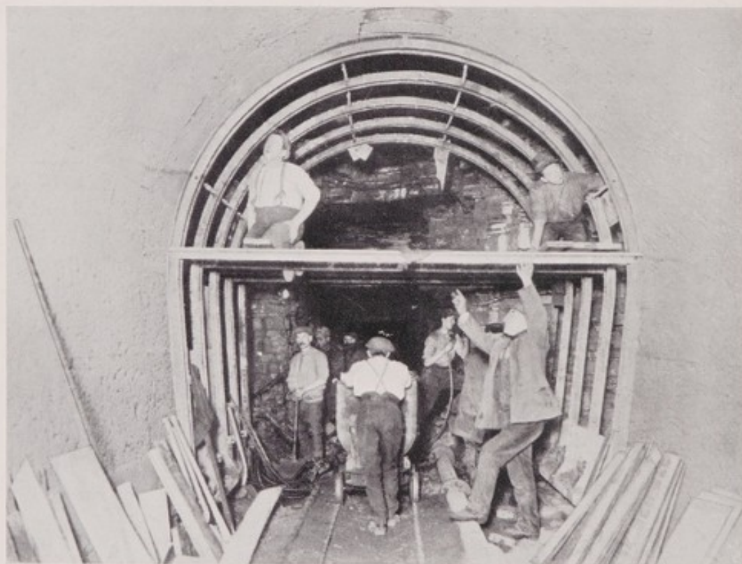
TUNNEL SEWER. CONCRETE LINING ON TRAVELLING STEEL CENTRES.
