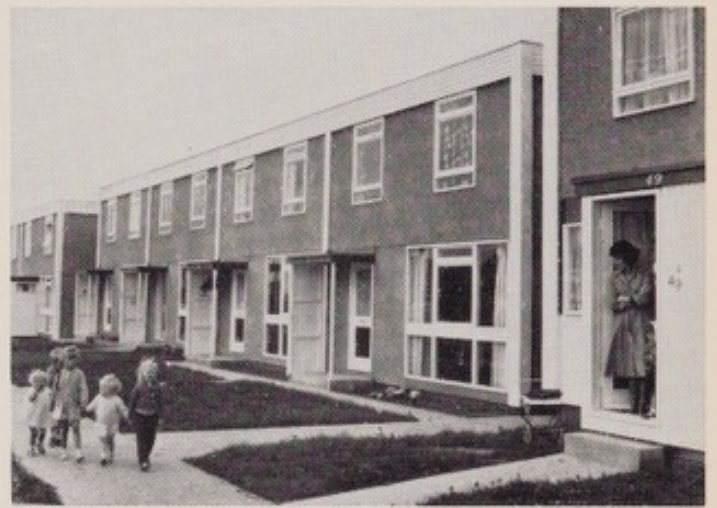
Prefabricated houses at Cramlington, Northumberland. Industrialised methods have the advantage of rapid construction and need fewer skilled workers.
