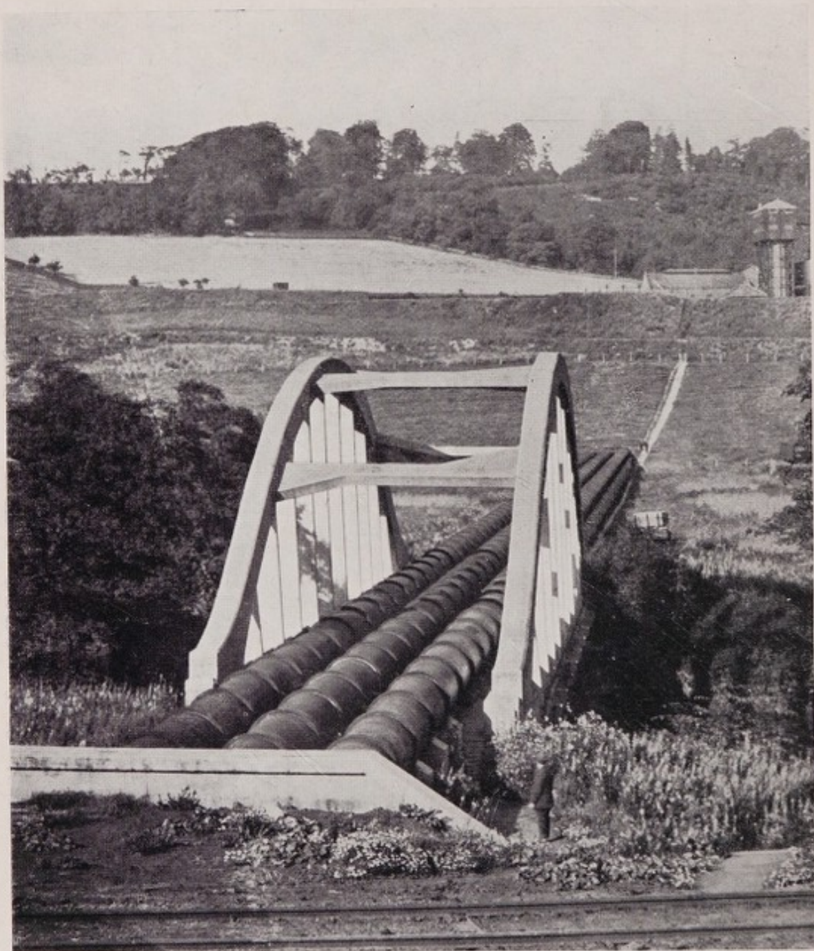
REINFORCED CONCRETE BRIDGE CARRYING SYPHON PIPE LINES
