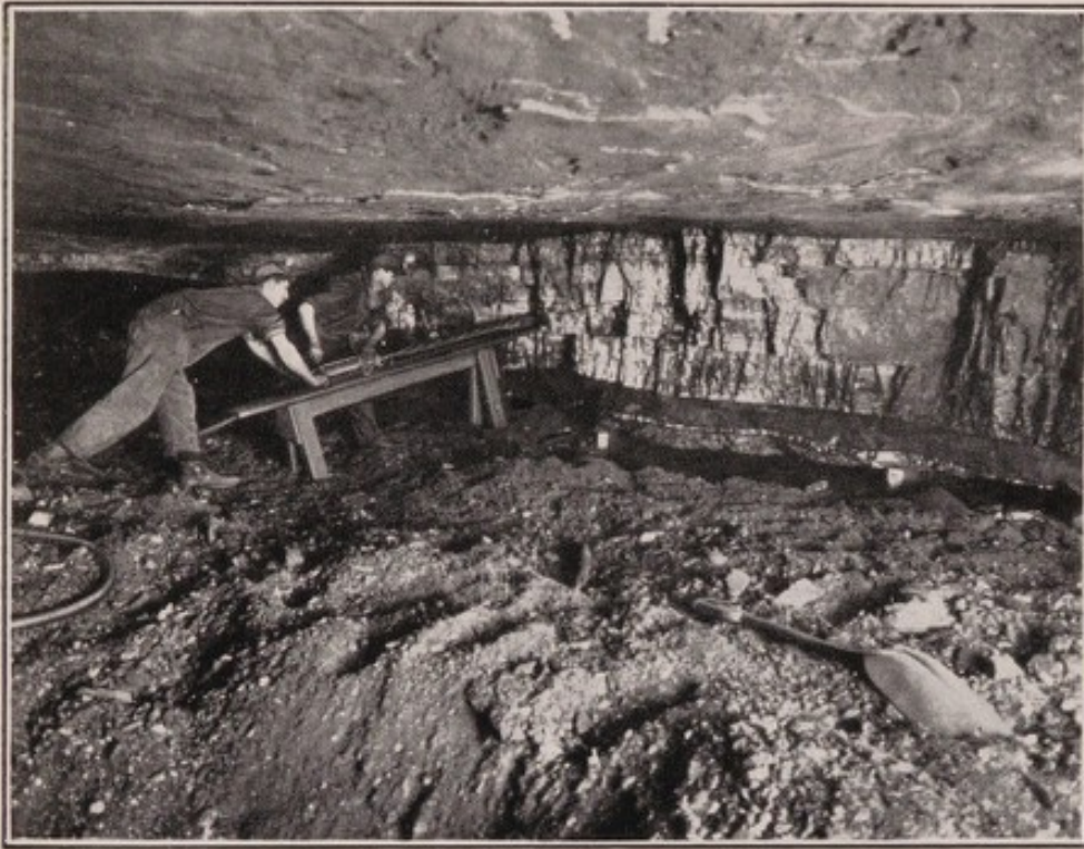
FIGURE 10.—DRILLING WITH JACKHAMMER.
