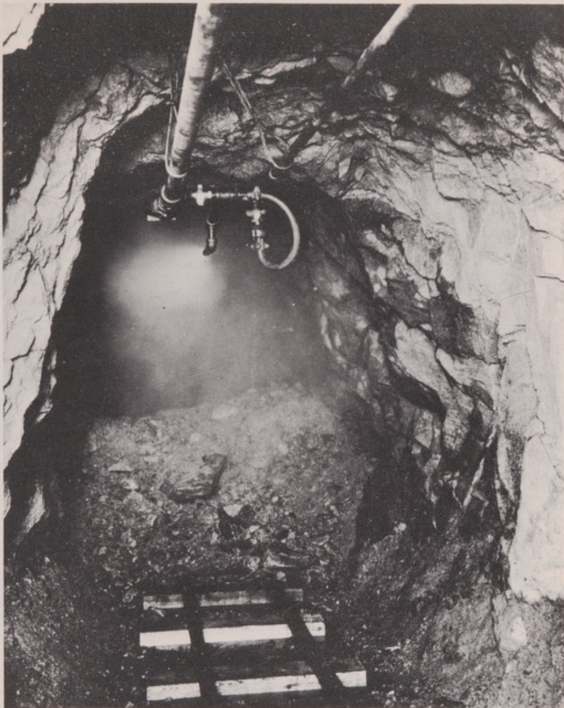
Compressed air and water mist spray used during blasting cycle in headings. (Courtesy of The Anaconda Co., 1963.)
