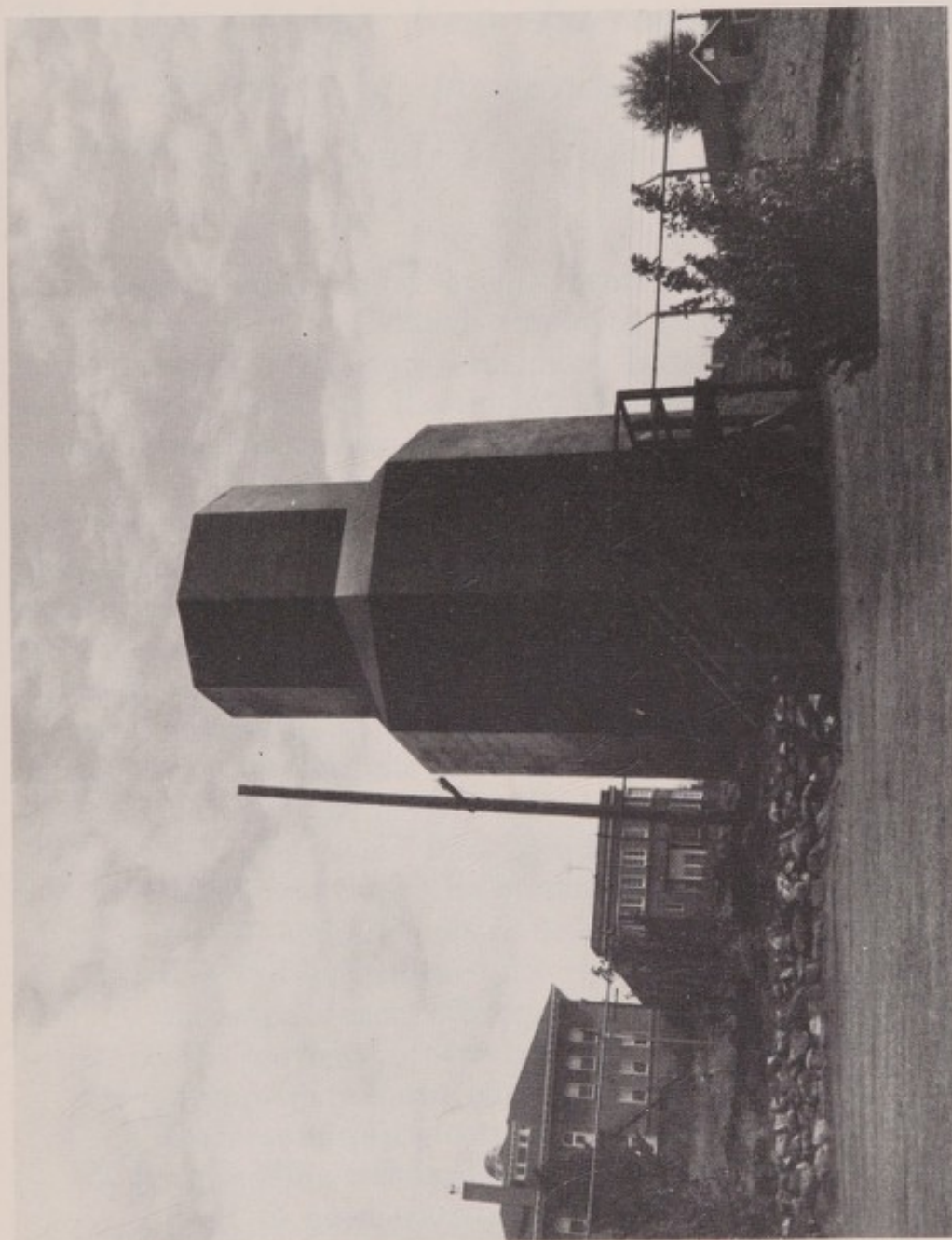
Air shaft discharge stack with acoustical lining to reduce noise. (Courtesy of The Anaconda Co., 1963.)
