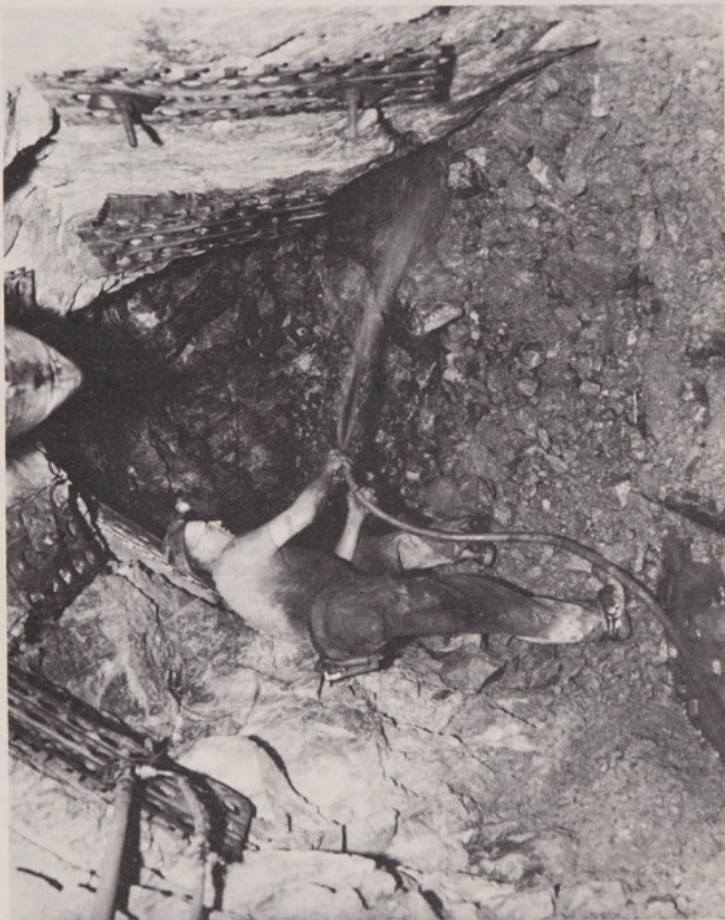
Miner wetting down muck pile and faces prior to mucking operation. Note overhead vent tubing and method of ground support. (Courtesy of The Anaconda Co., 1963.)
