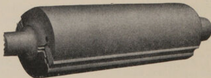
FIG. 51 E.—2-Cutter Circular Block. Note the "back irons." (Messrs. A. Ransome & Co., Ltd., Newark-on-Trent.)
