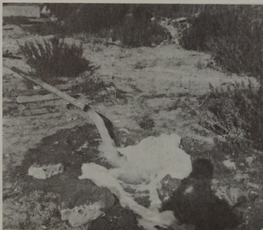
Foam from test well No. 2 during development.
