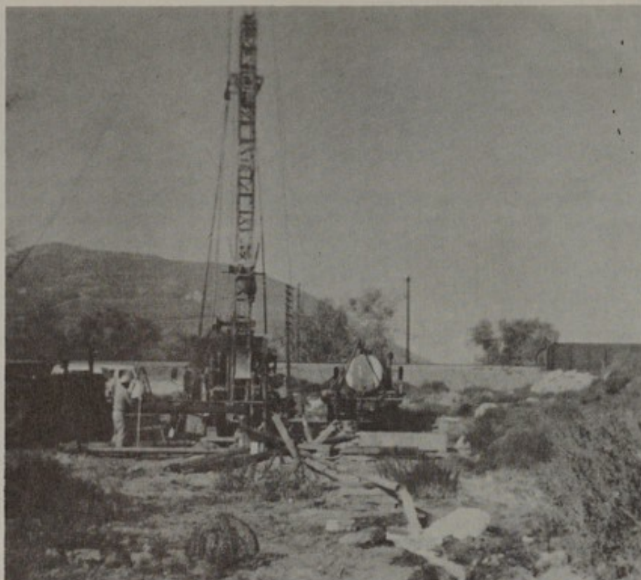
Construction of test well No. 2.
