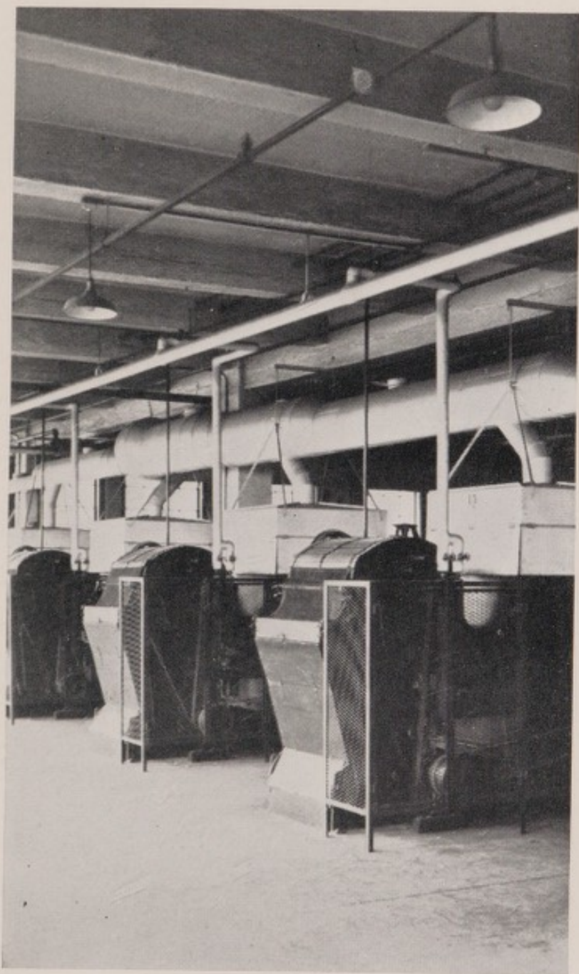
FIGURE 24.—HOODS USED ON GERMAN-TYPE BLOWING MACHINES.
