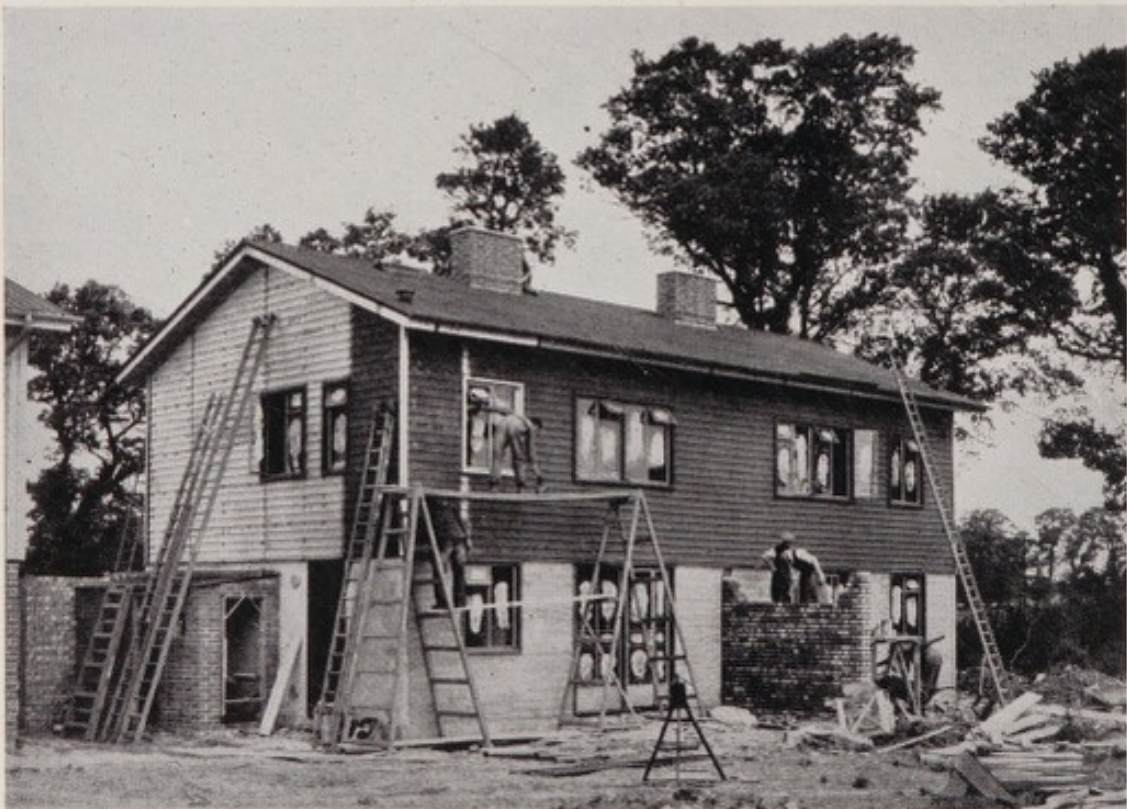
Meanwhile, Block 12 has also been making good progress. The ground floor brick cladding is nearly up and the chimney cappings are being fixed. Both houses are nearly ready. (Fig. 29.)
