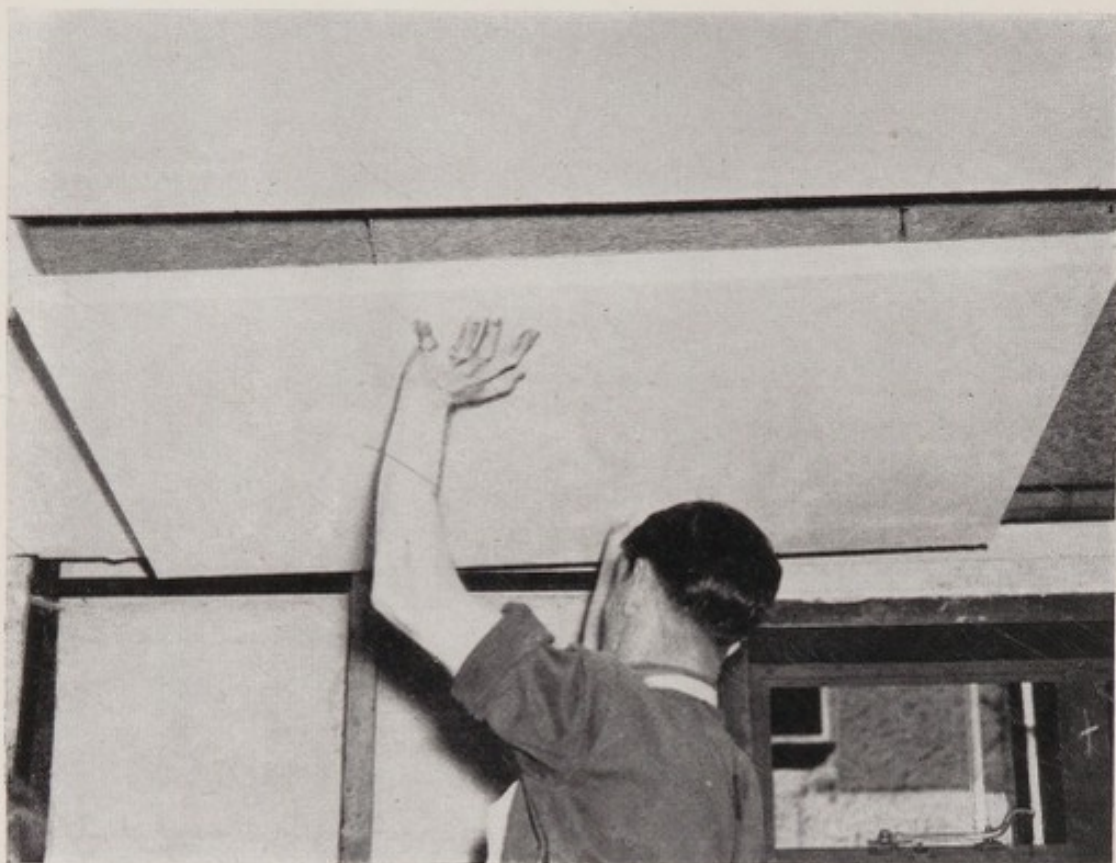
Below the wood wool mats (see Fig. 12) prefabricated ceiling slabs of plasterboard are slid into position. The slabs are 4 ft. long. (Fig. 15.)
