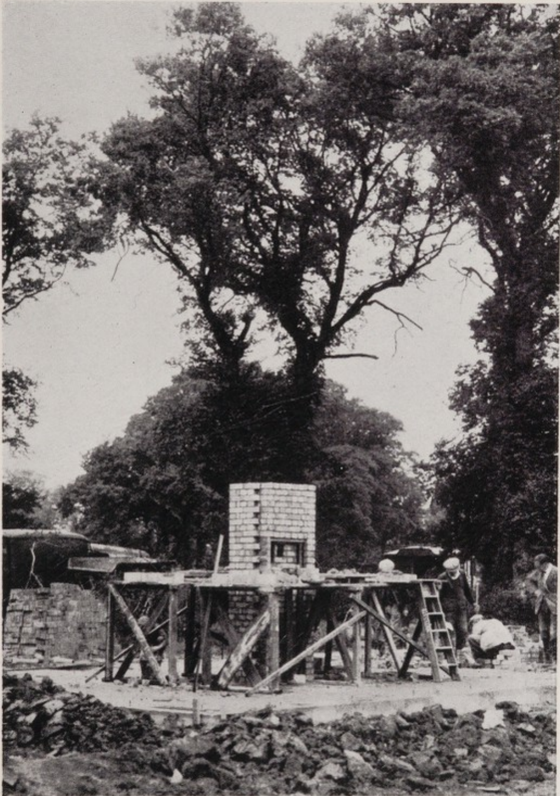
With this house, once the site concrete is down, the next job is to start the building of the brick flue stacks. (Fig. 23.)
