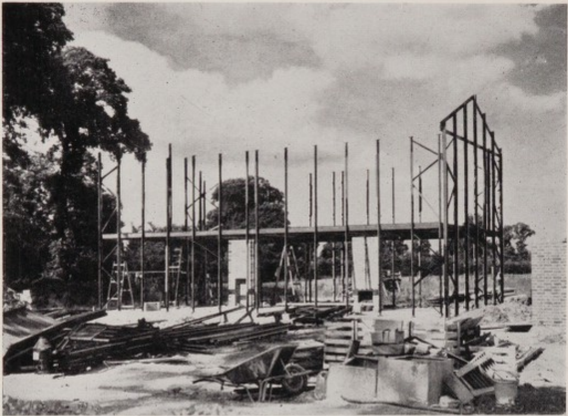
Stacks and frame go up together. After four days, the posts are in position complete with corner braces. One of the gables has been erected. (Fig. 24.)
