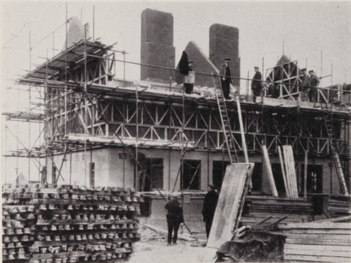
Fourteen days later this shuttering has done its work and can be struck. The first floor shuttering will be the last to come down. (Fig. 36.)
