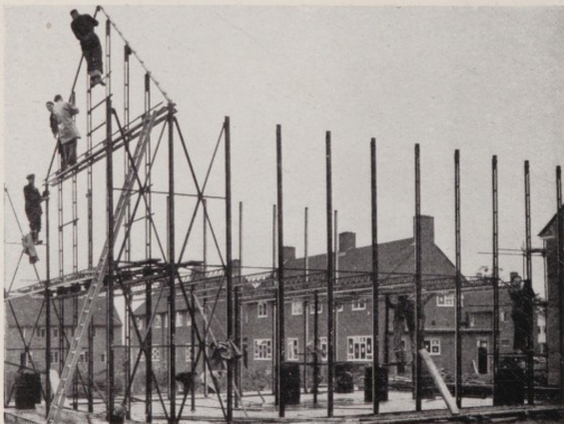
After half a day's work on the steel frame, the men on the left are completing the party wall framing. Stiffening braces are used on each side of the party wall. (Fig. 6.)
