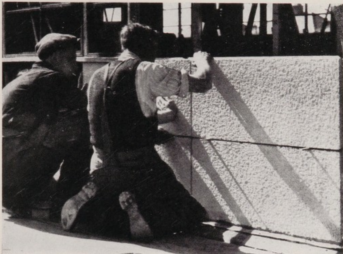
The external wall slabs are 3 ft. 4 ins. long, 1 ft. 4 ins. wide. They are made of pressed vibrated concrete, 2 ins. thick, into which a coloured rendering has been cast. (Fig. 13.)
