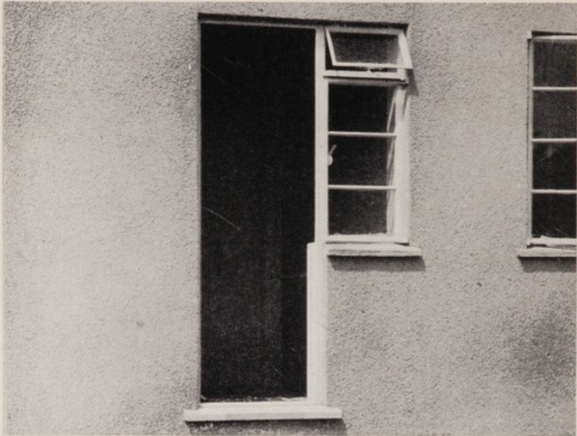
A clear, even colour penetrates into the deeply textured wall. The plinth rendering is applied by hand in the usual way. (Fig. 39.)
