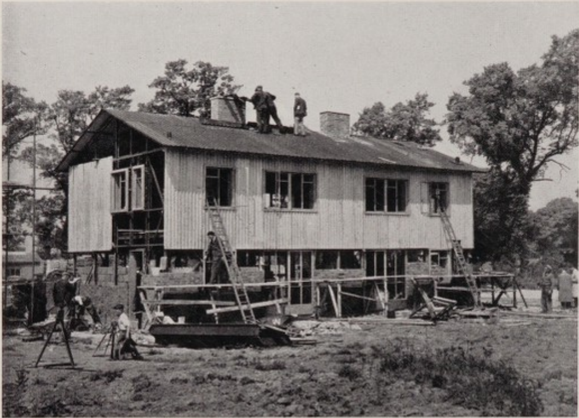
Meanwhile, Block 12 has also been making good progress. The ground floor brick cladding is nearly up and the chimney cappings are being fixed. Both houses are nearly ready. (Fig. 29.)
