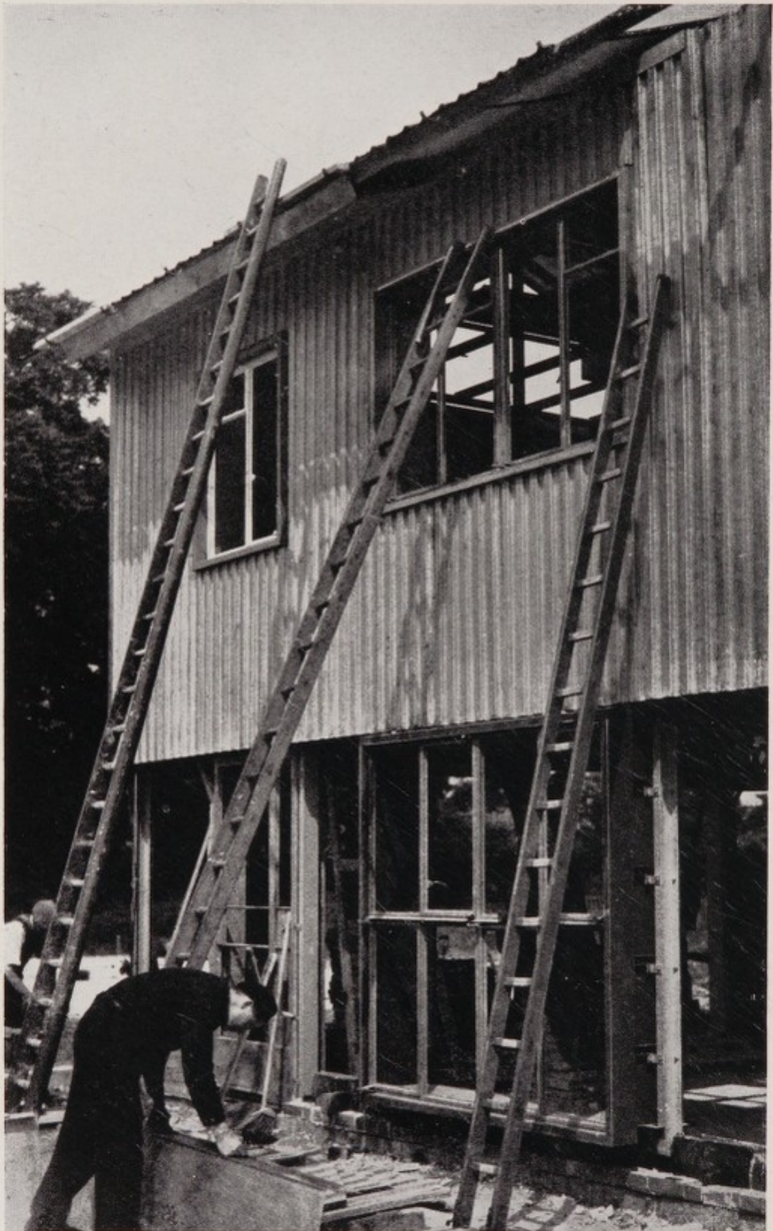
In Block 12, the vertical rib steel cladding to the first floor is completed. Eaves and fascia units are being fixed. The bricklayers are about to start on the ground floor cladding. (Fig. 27.)
