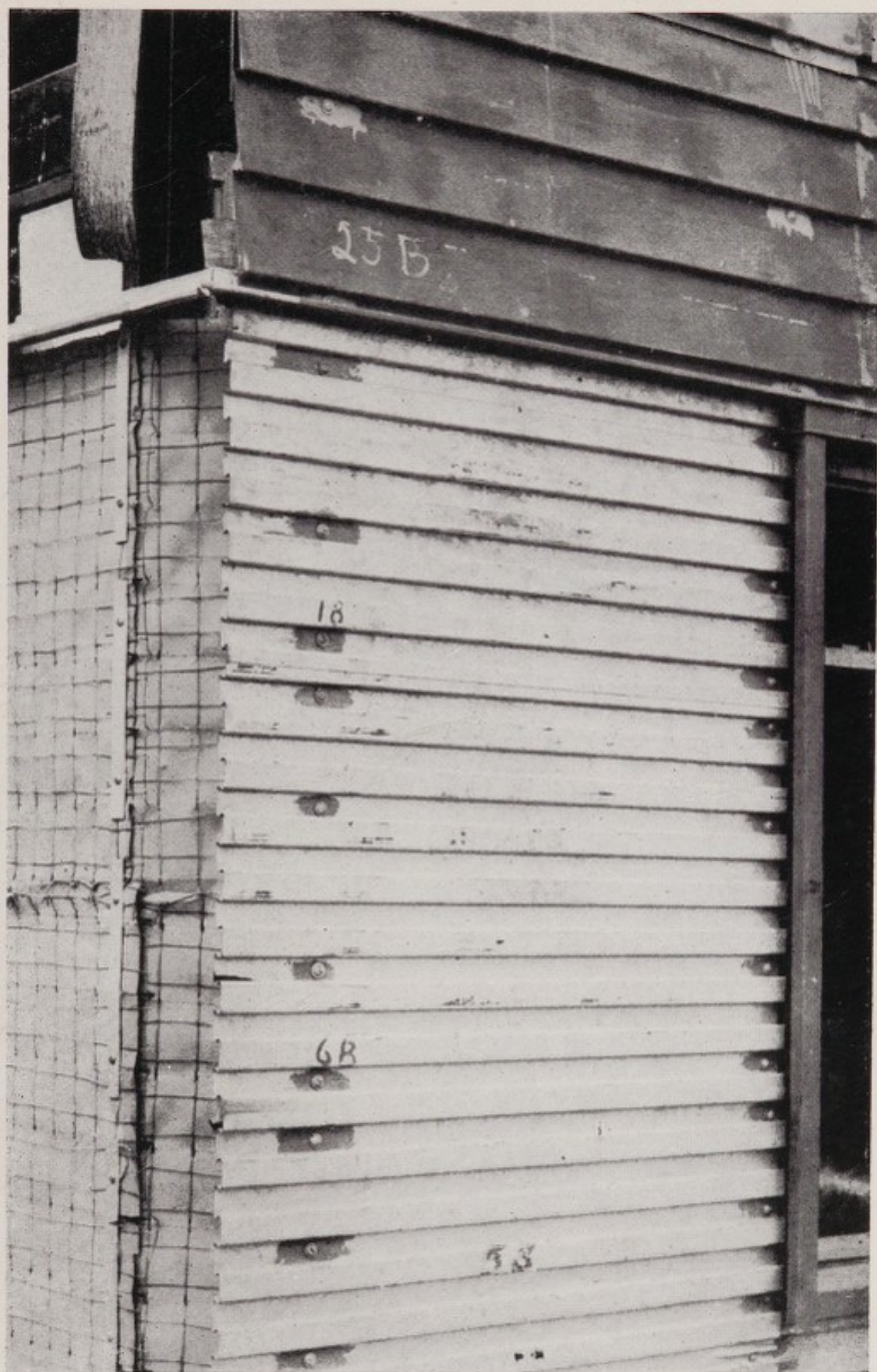
The ground floor of Block 13 has steel cladding to back and front walls, dovetailed to hold the rendering. The rendering on the end walls goes on a wire mesh fabric backed with building paper. (Fig. 28.)
