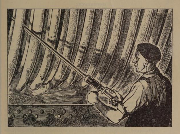
Fig. 16. Tube cleaning by percussion lance.
