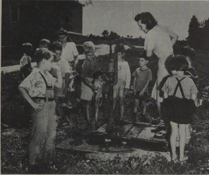
This leaky wooden pump platform leaves the well open to contamination which may infect all the pupils in the school.
