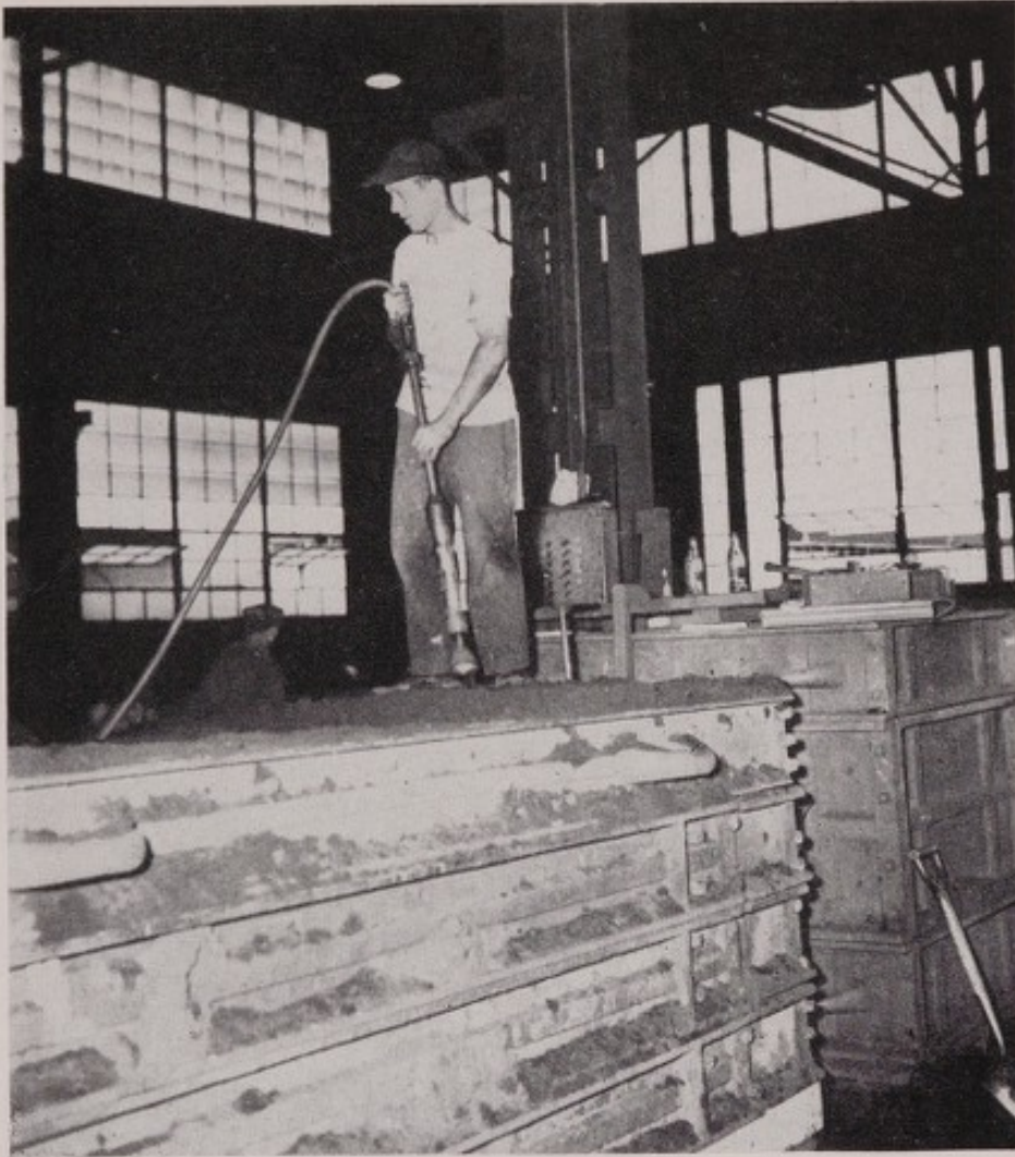
Figure 1.—Tamping sand into a large floor mold with a pneumatic tool. Note the large window space which aids in providing natural ventilation and illumination.
