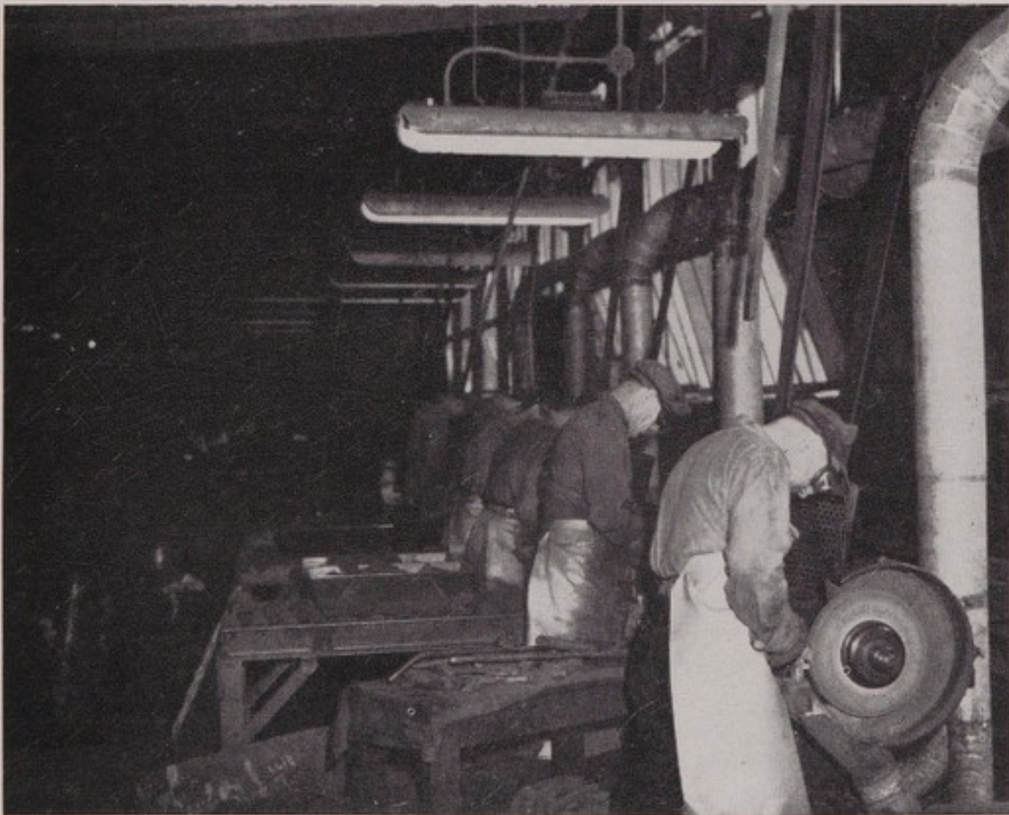
Figure 7.—Stand (stationary) grinding small castings. Note fluorescent lights and ducts of exhaust ventilation system.
