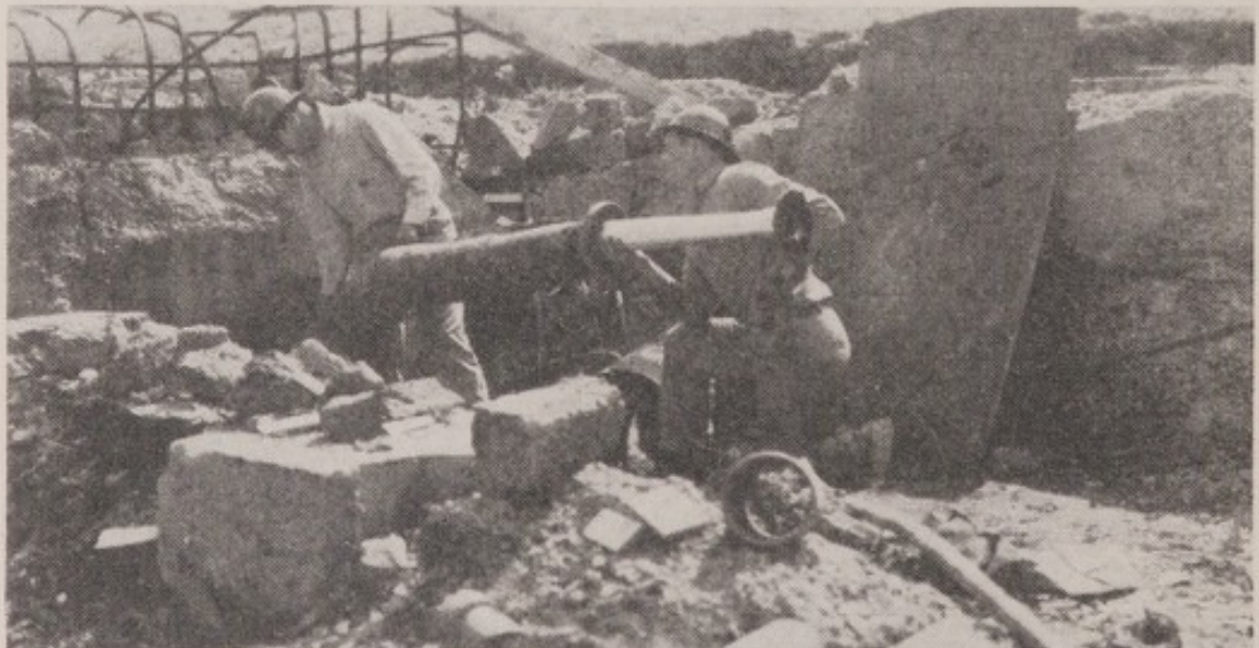
FIGURE 12.—Improved ventilation. Use of flexoid tubing in connection with air-mover. Tubing being extended to working face by workman (underground) using oxygen-breathing apparatus.
