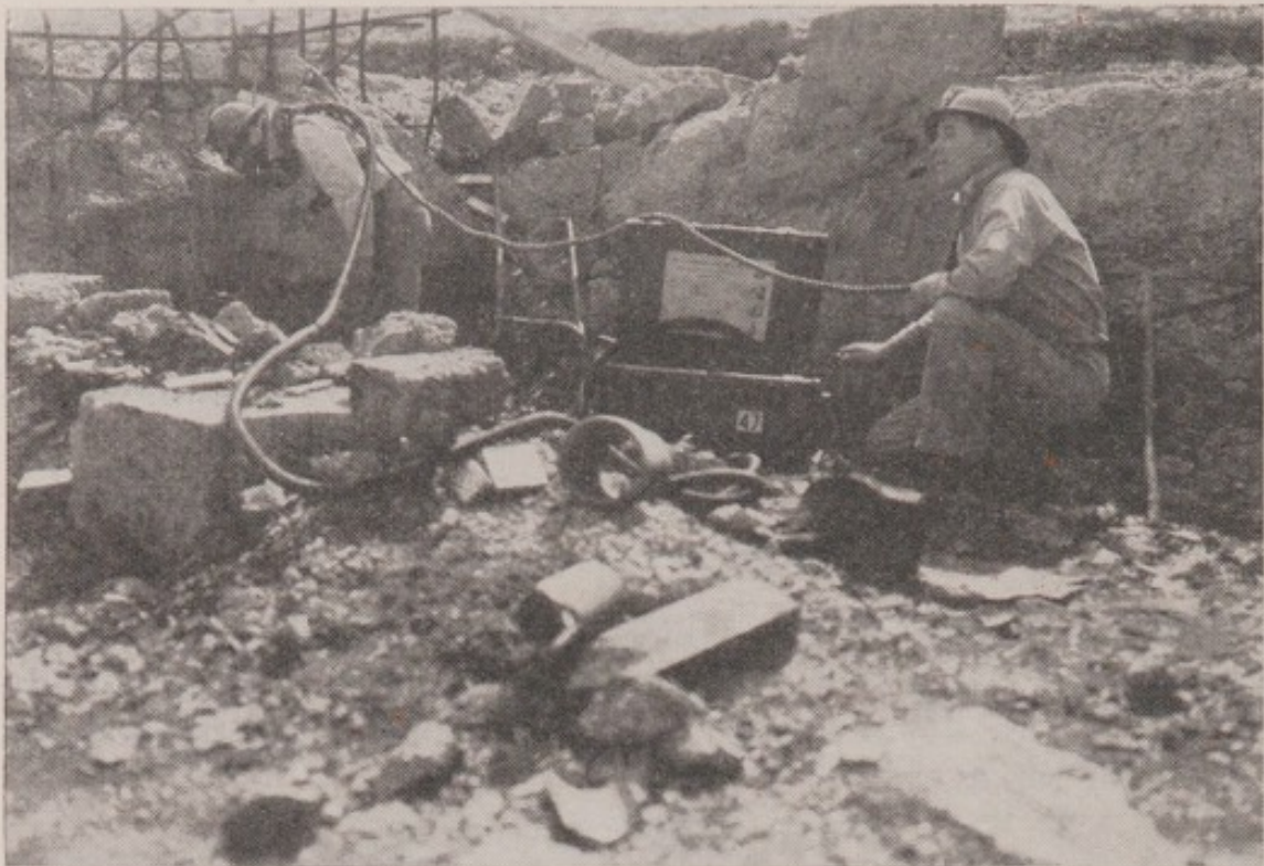
FIGURE 38.—Hose mask equipped with blower and life line. Wearer about to explore opening under pile of debris.
