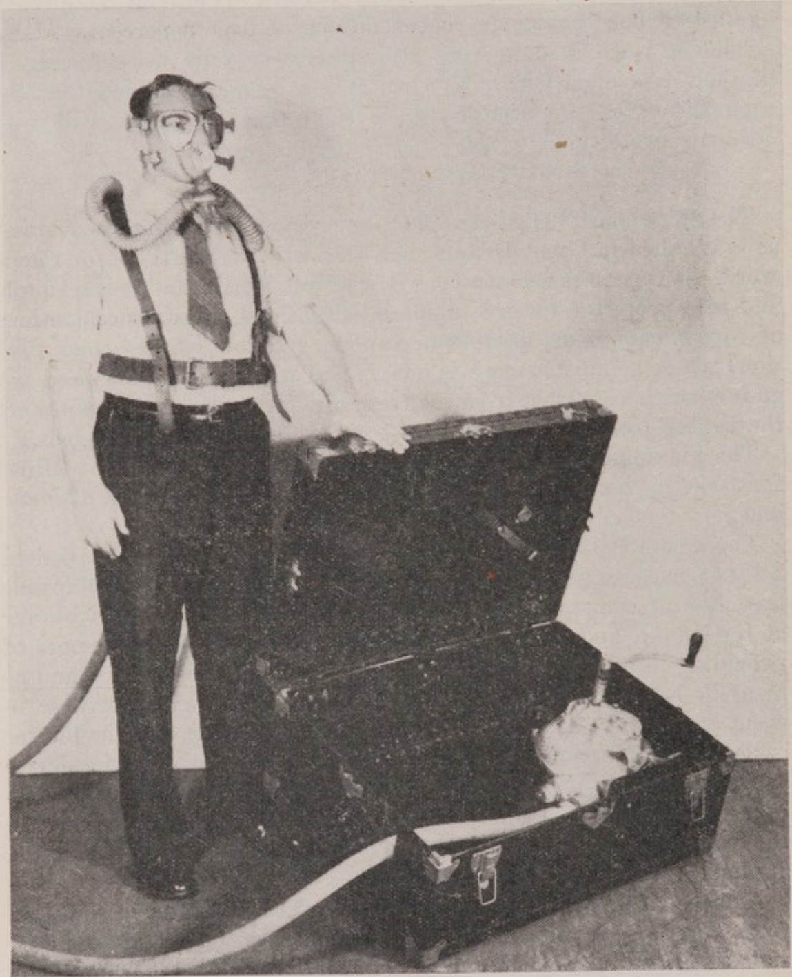
FIGURE 3.--Hose mask and blower.
