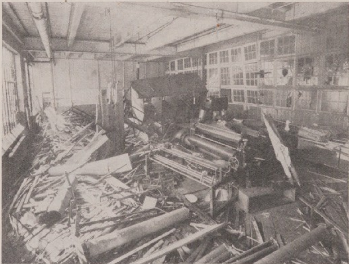
FIGURE 37.—Damage caused by an explosion of about 600 cubic feet of utility gas-air mixture, leaking in from old buried abandoned gas service pipe.
