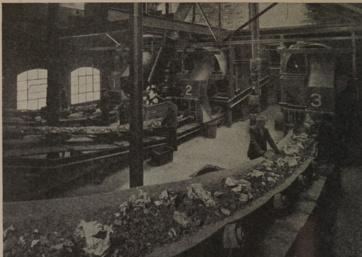
FIG. 48.—View of picking belts, Brookvale Road Depot, Birmingham.
