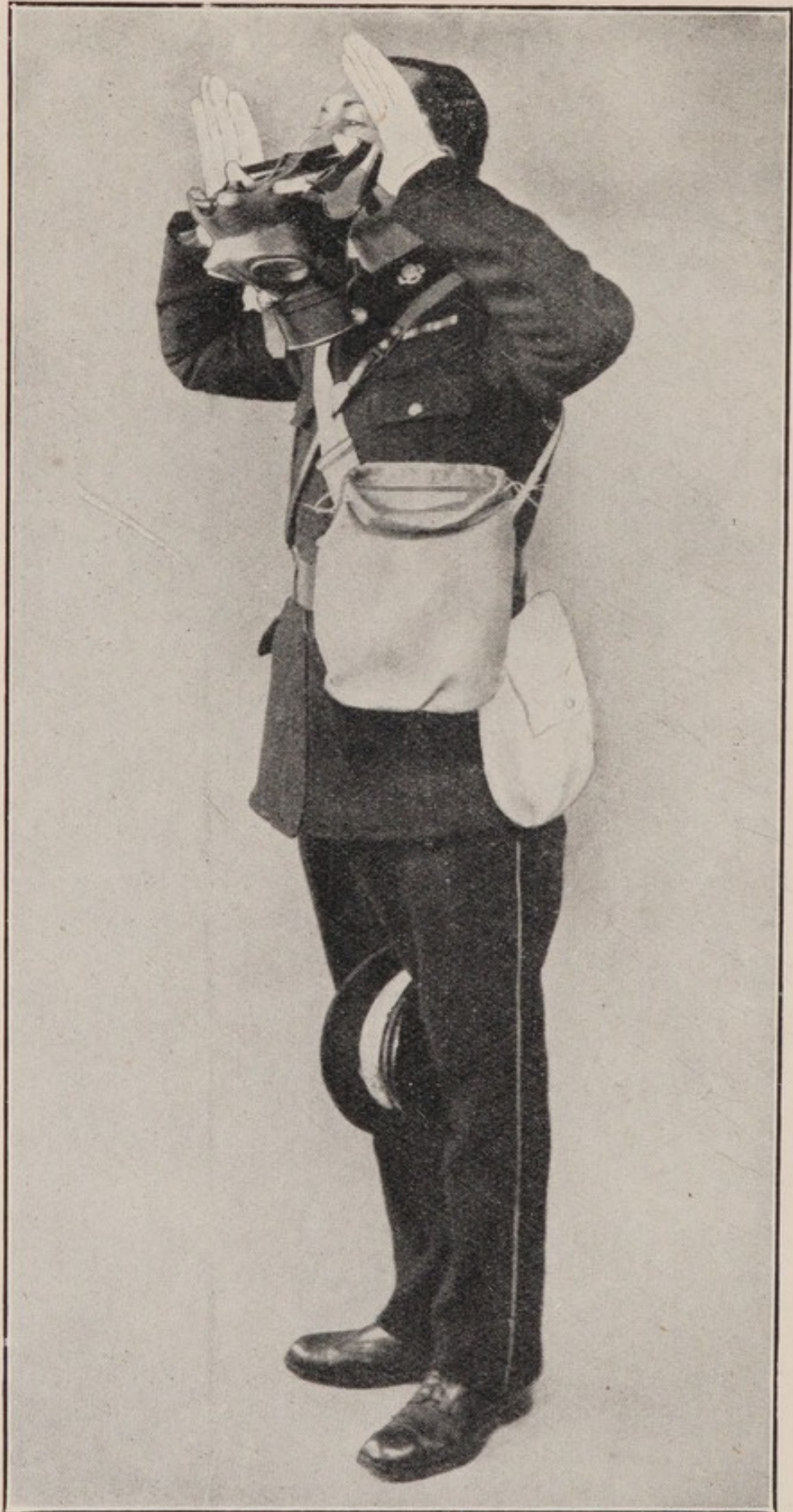
FIG. 16—CIVILIAN DUTY RESPIRATOR—ACTION ON ALARM "GAS", STAGE THREE.
