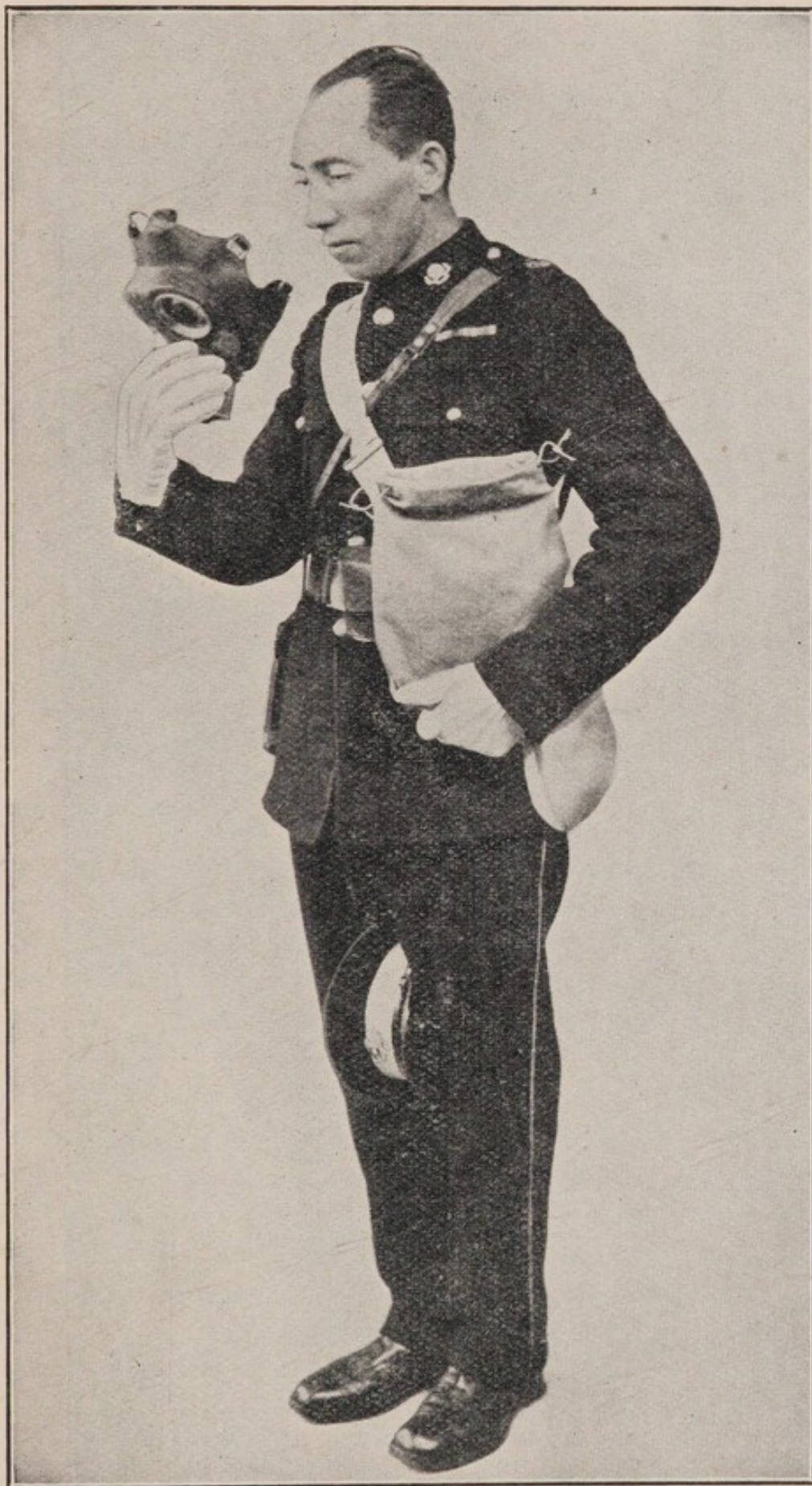
FIG. 15—CIVILIAN DUTY RESPIRATOR—ACTION ON ALARM "GAS", STAGE TWO.
