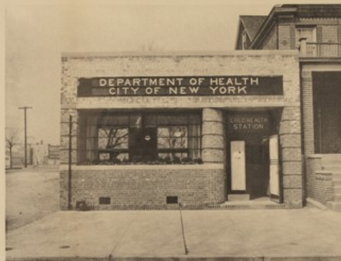
Photograph of New, Modern Fireproof, Well-Lighted and Ventilated Child Health Station Building
