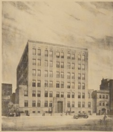
TYPICAL DISTRICT HEALTH CENTER DEPARTMENT OF HEALTH - CITY OF NEW YORK
