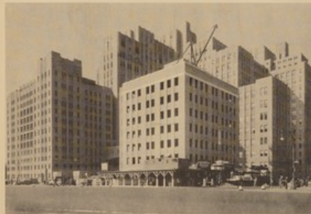
WASHINGTON HEIGHTS HEALTH & TEACHING CENTER COLUMBIA PRESBYTERIAN HOSPITAL, 2150 W. 185th STREET FOR THE DEPARTMENT OF HEALTH, CITY OF NEW YORK
