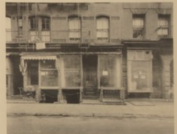
Unsatisfactory Quarters in an Obsolete Tenement
