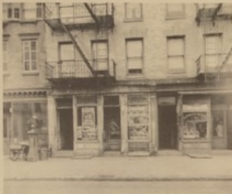
A Dark Store Poorly Heated and Ventilated
