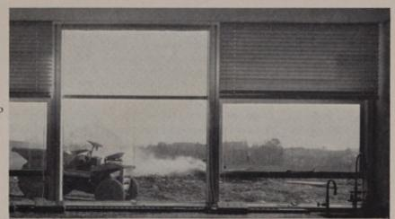
(e) Roller blinds. The materials used in roller blinds may be either the traditional holland, or, as in the photograph, a woven plastic giving the correct transmission factor (paragraph 93).
