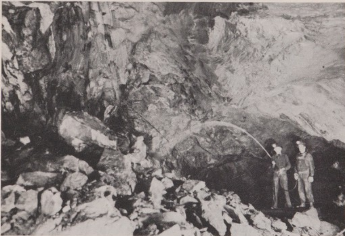
FIGURE 10.—Watering in Shrinkage Stope.
