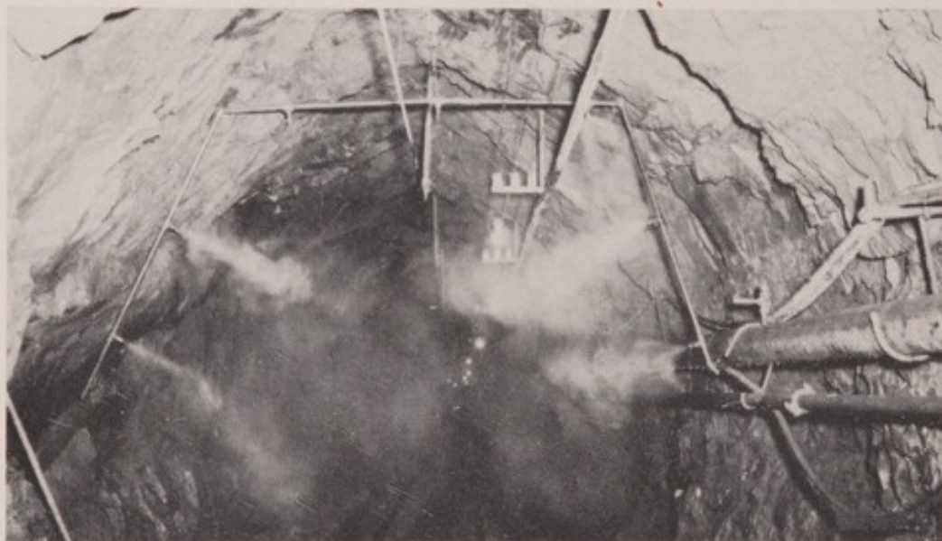
FIGURE 8.—Water Curtain in Drift.
