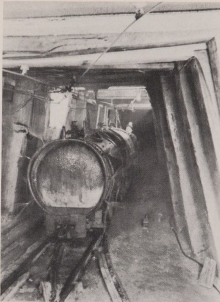
FIGURE 6.—Fine-Spray Nozzles on Tank Car.
