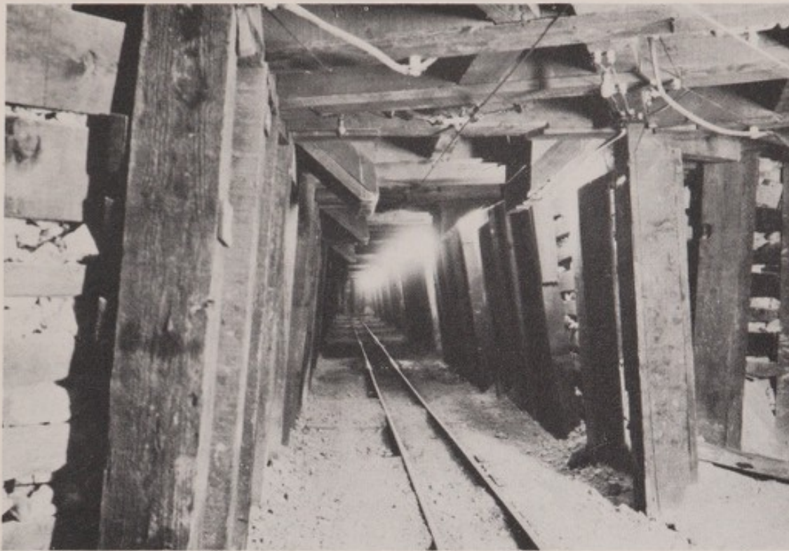
FIGURE 36.—Lighting in Timbered Haulageway.
