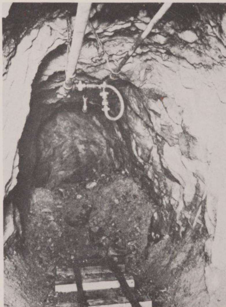
FIGURE 12.—Air-Water Spray at Face of Drift.
