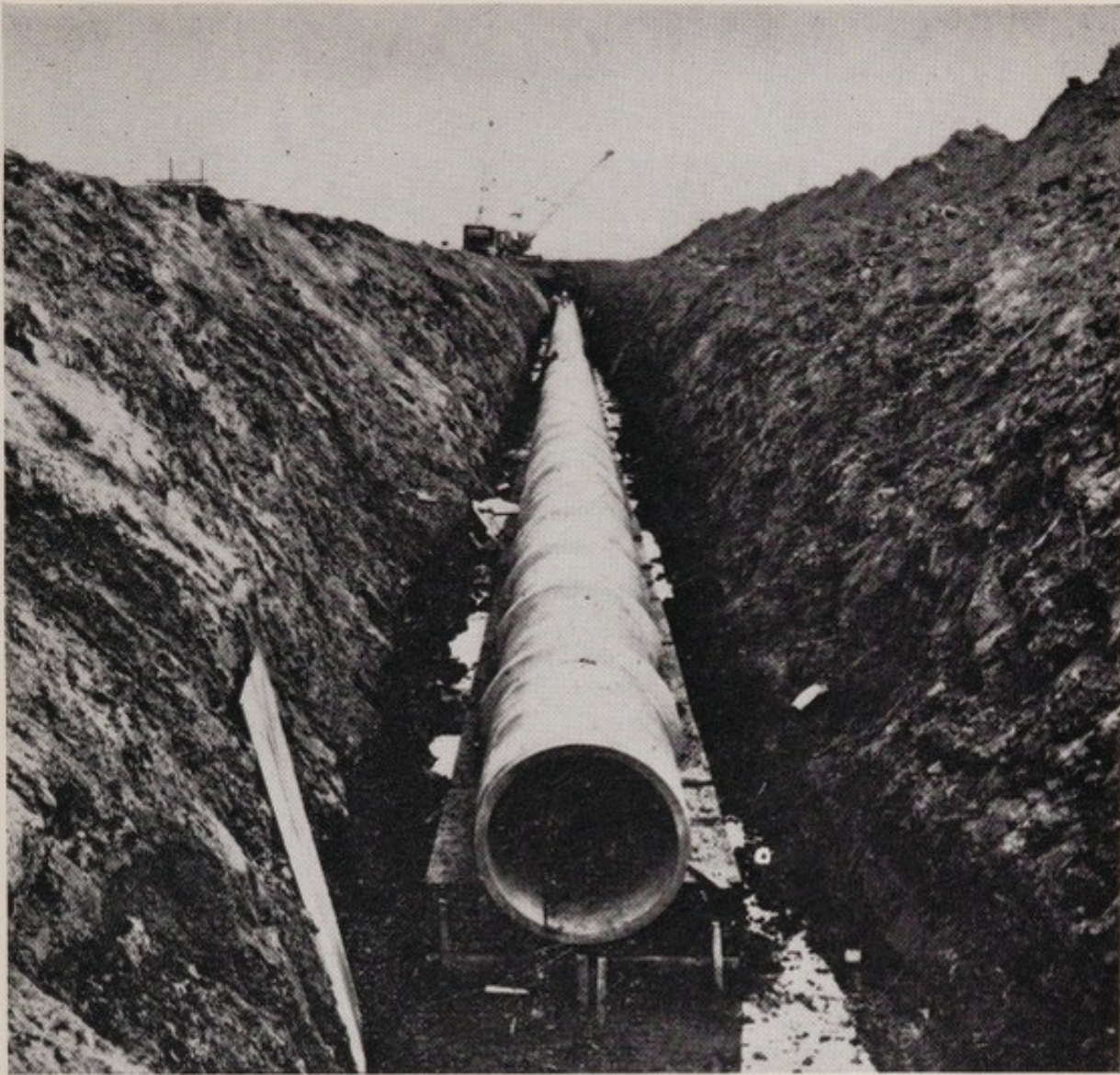
5. A pre-cast concrete pipe sewer laid in battered trench excavation
