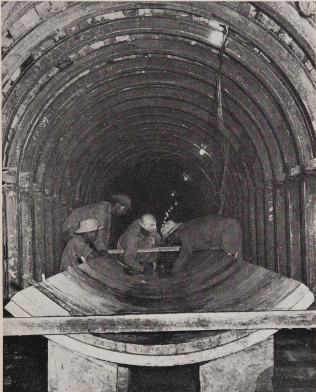
7. Construction of a 72-inch (183 cm) diameter sewer in heading at Singapore
