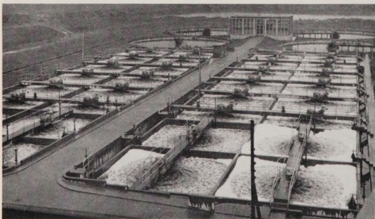
28. Simplex High Intensity Cones treating industrial sewage at the Aldwarke Works of the County Borough of Rotherham
