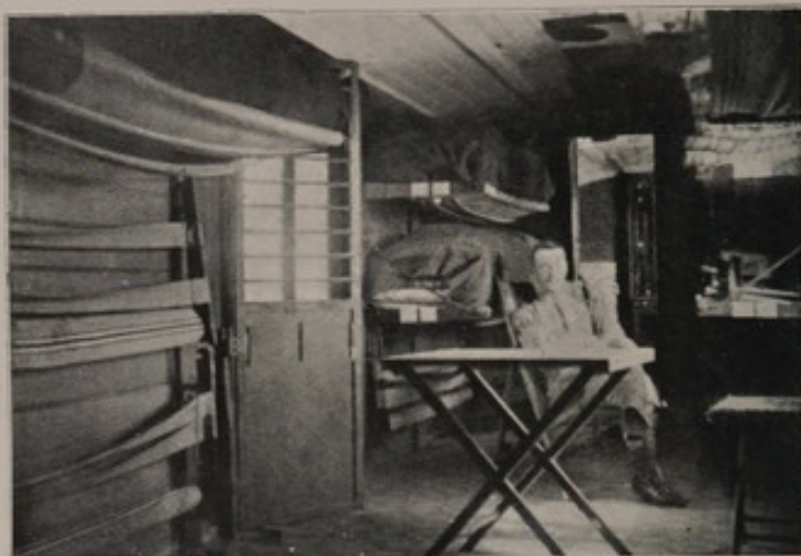
NO. 4 AMBULANCE TRAIN. (Showing method of folding up cots.)
