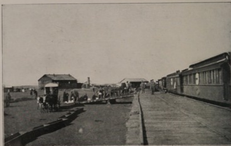
HOSPITAL SIDING AND PLATFORM AT SPRINGFONTEIN. (Unloading No. 5 Ambulance Train.)
