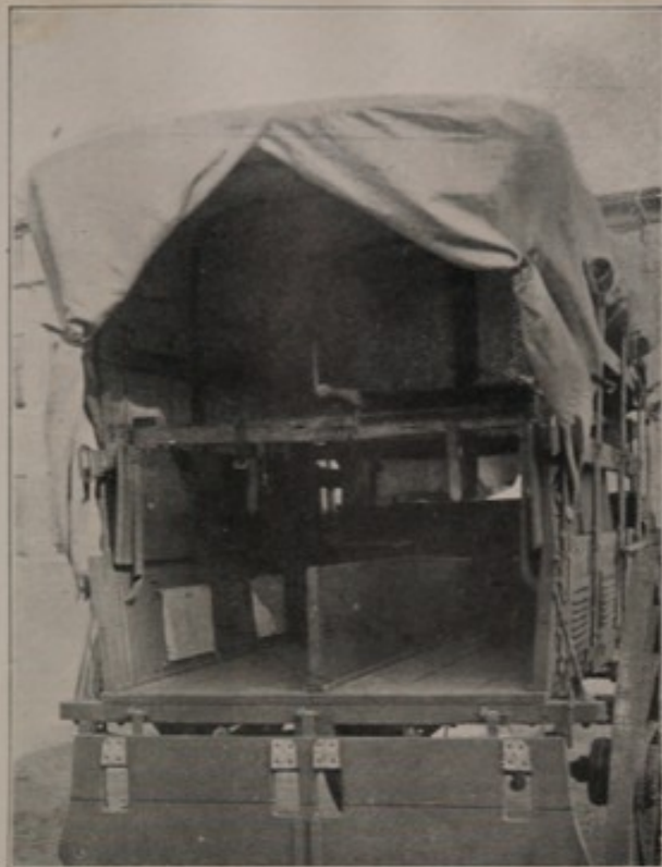
MARK V AMBULANCE. (Converted to carry four cases. Captain Stammer's method.)
