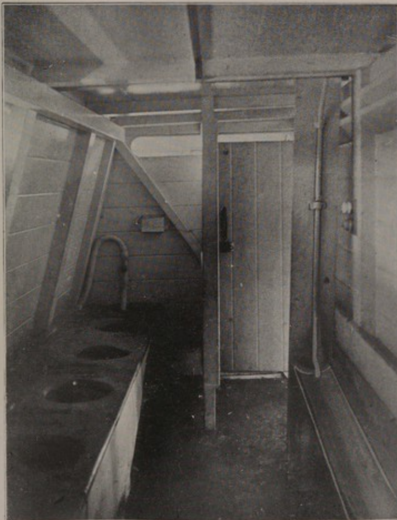
NO. 1, PART OF TROOP LATRINE SHOWING URINAL ON RIGHT OF PHOTO.
