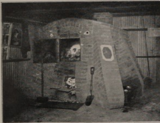
INCINERATOR. NO. 20 GENERAL HOSPITAL.
