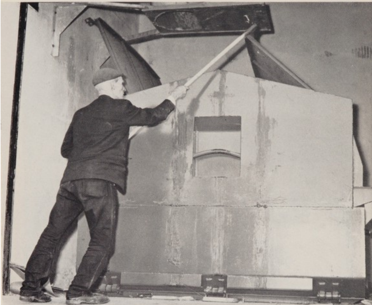
11. A large capacity interchangeable container serving a refuse chute
