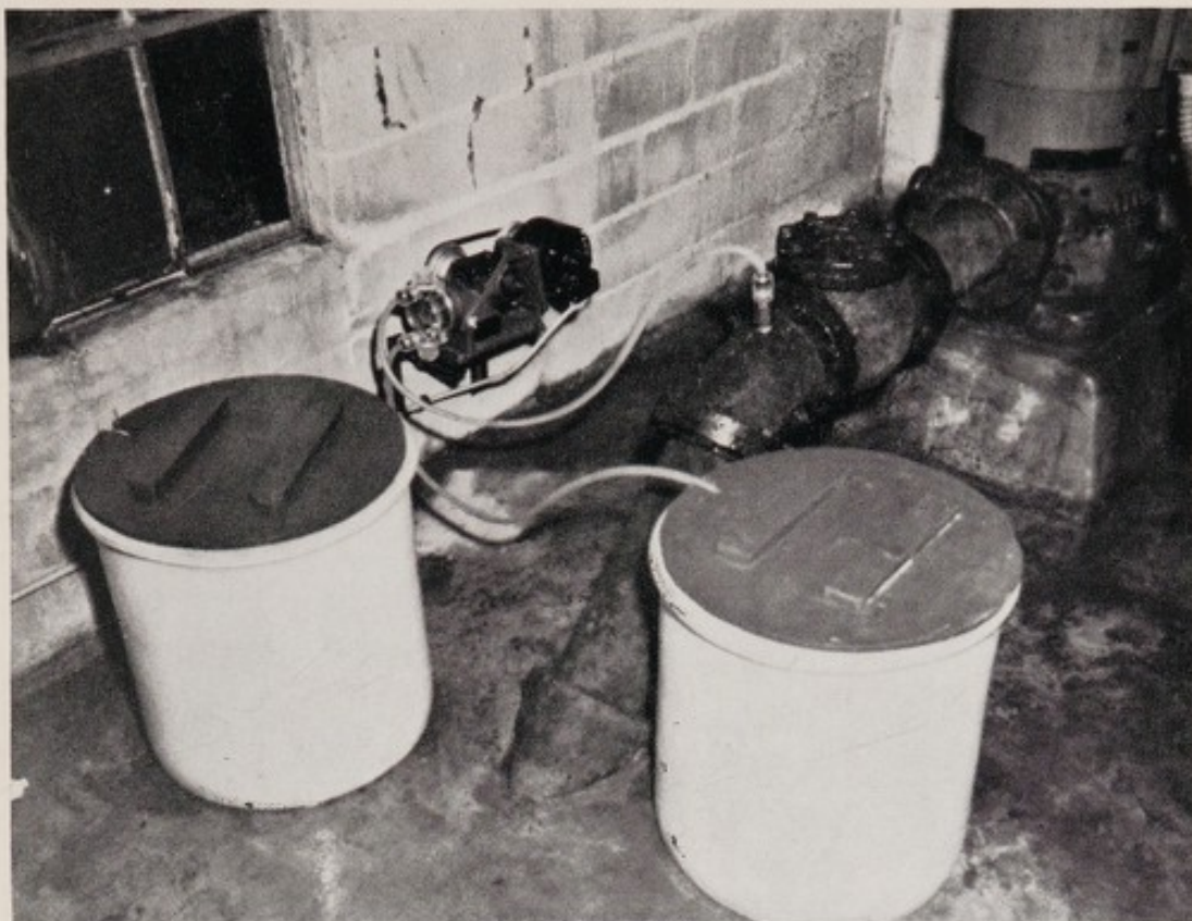
PLATE 1 Solution feed of sodium fluoride. Proportioneer feeder. Crestwood, Wis.
