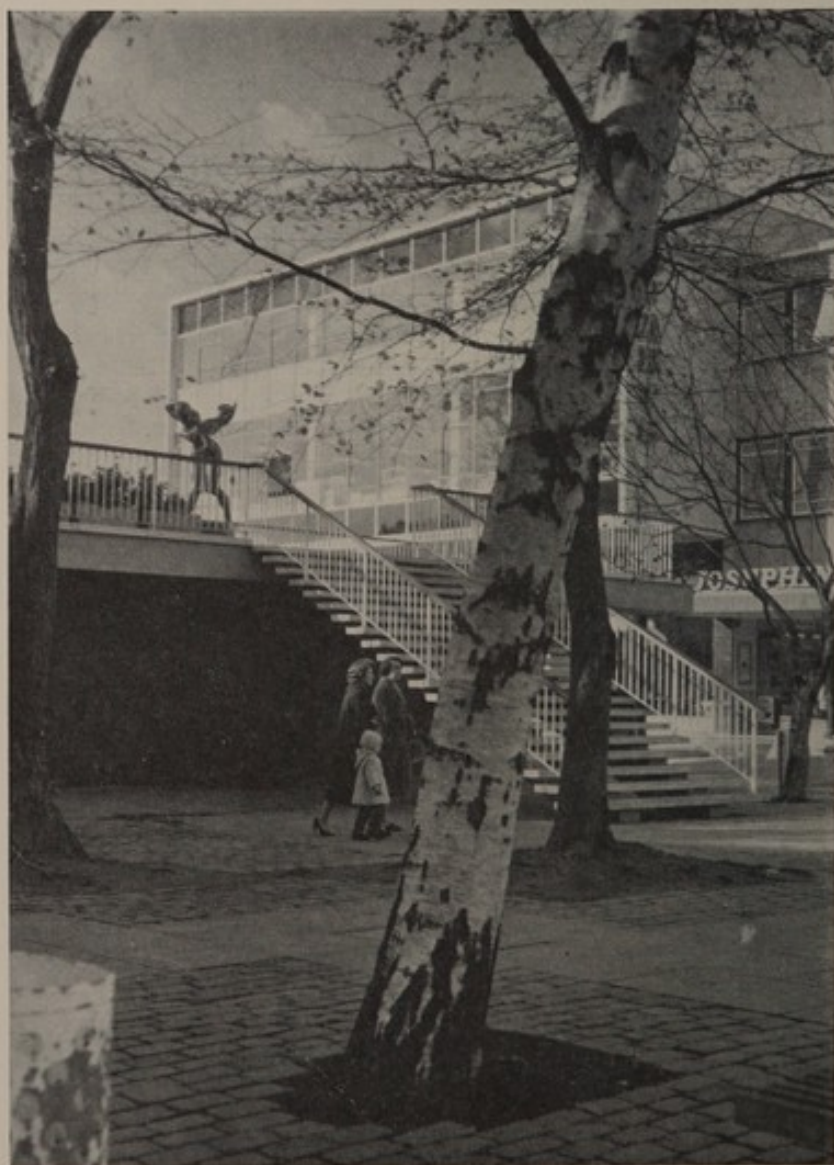
211 The pedestrian centre at Stevenage New Town.
